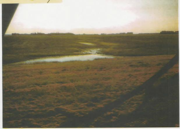
Looking from top of dike down to field. This is one of the places where there is seepage underneath the dike of the diversion. In this case it came to the surface and pooled because of blocked ditches.
