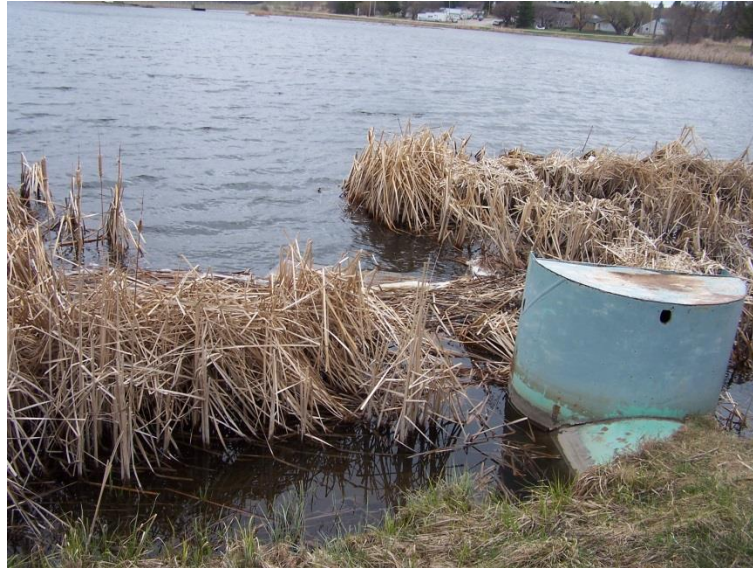
Figure A5-3 View of the fish ladder inlet on the Rapid City Reservoir side with small area of cattail immediately in front of the opening, April 25, 2012.
