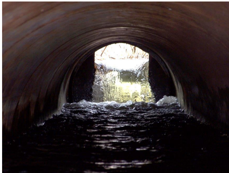
Figure A5-2. View of the 0.3 m water level differential between the inside of the fish ladder culvert and the Rapid City Reservoir, April 25, 2012.
