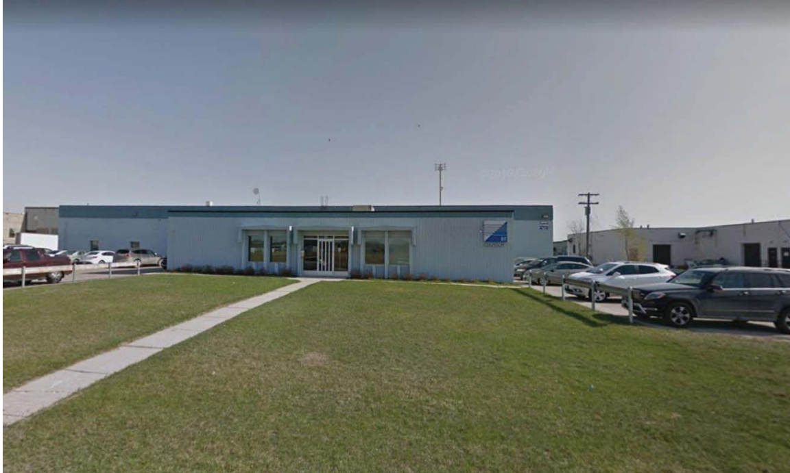
Photo B-1: B/E Aerospace building facing north and adjacent parking areas
