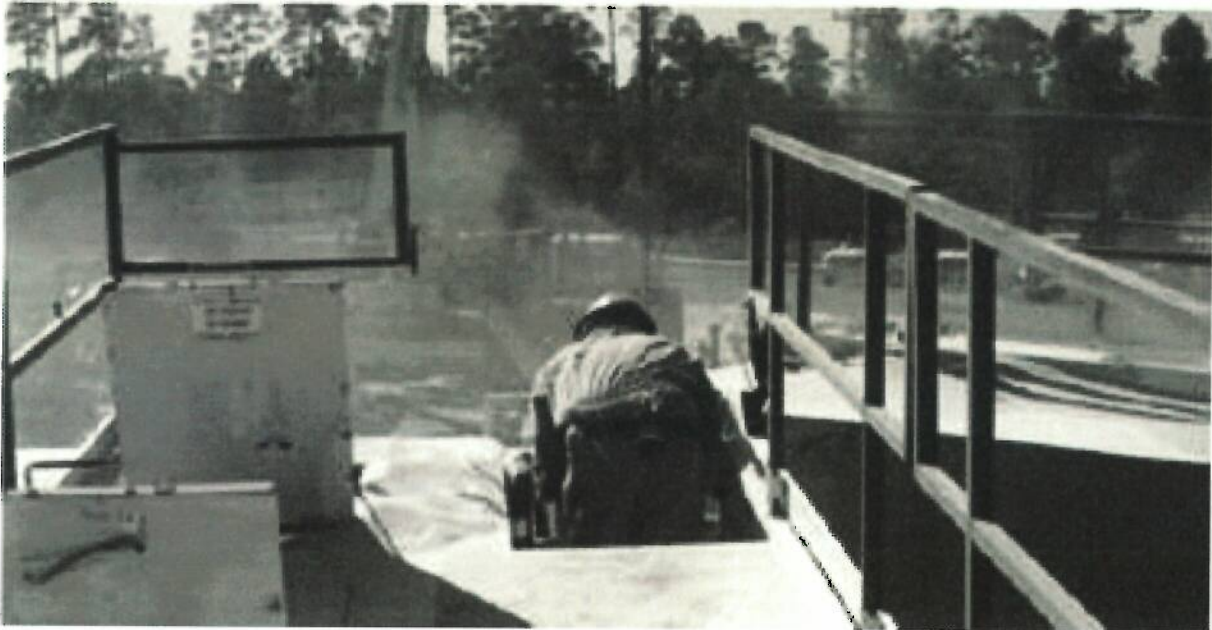
Figure 8 Worker exposure to dust from thief hatches
