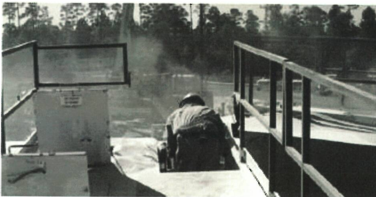
Figure 8 Worker exposure to dust from thief hatches
