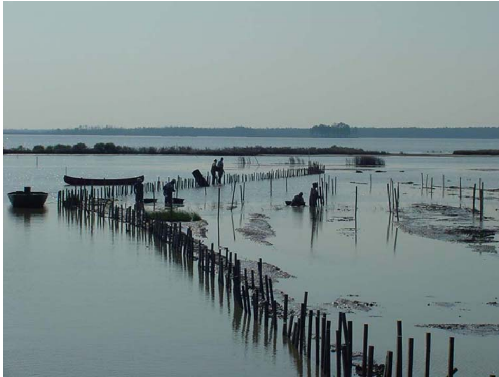
Installation of straw bales using posts in a shallow marsh environment.
