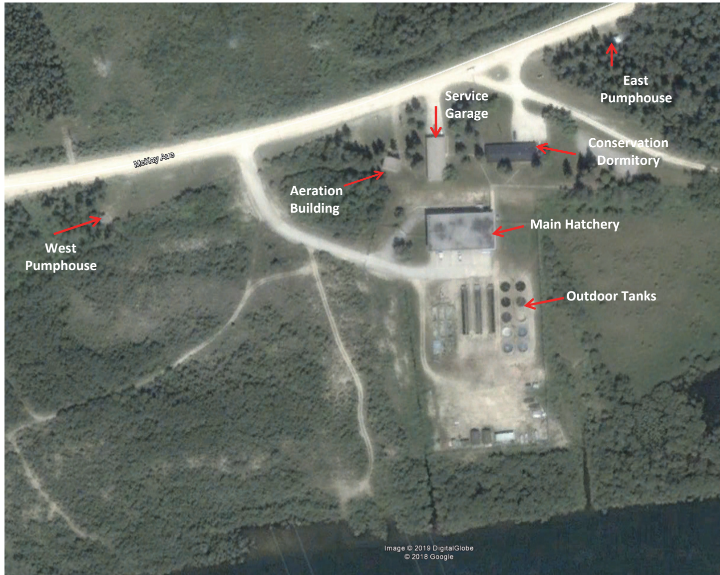
Figure 2: Aerial view of the Grand Rapids Fish Hatchery
