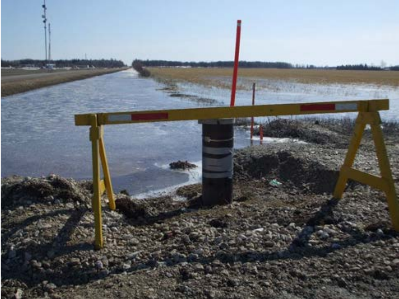
Figure 7. Flooding of ditch and adjacent field, encroaching on West well casing in foreground.
