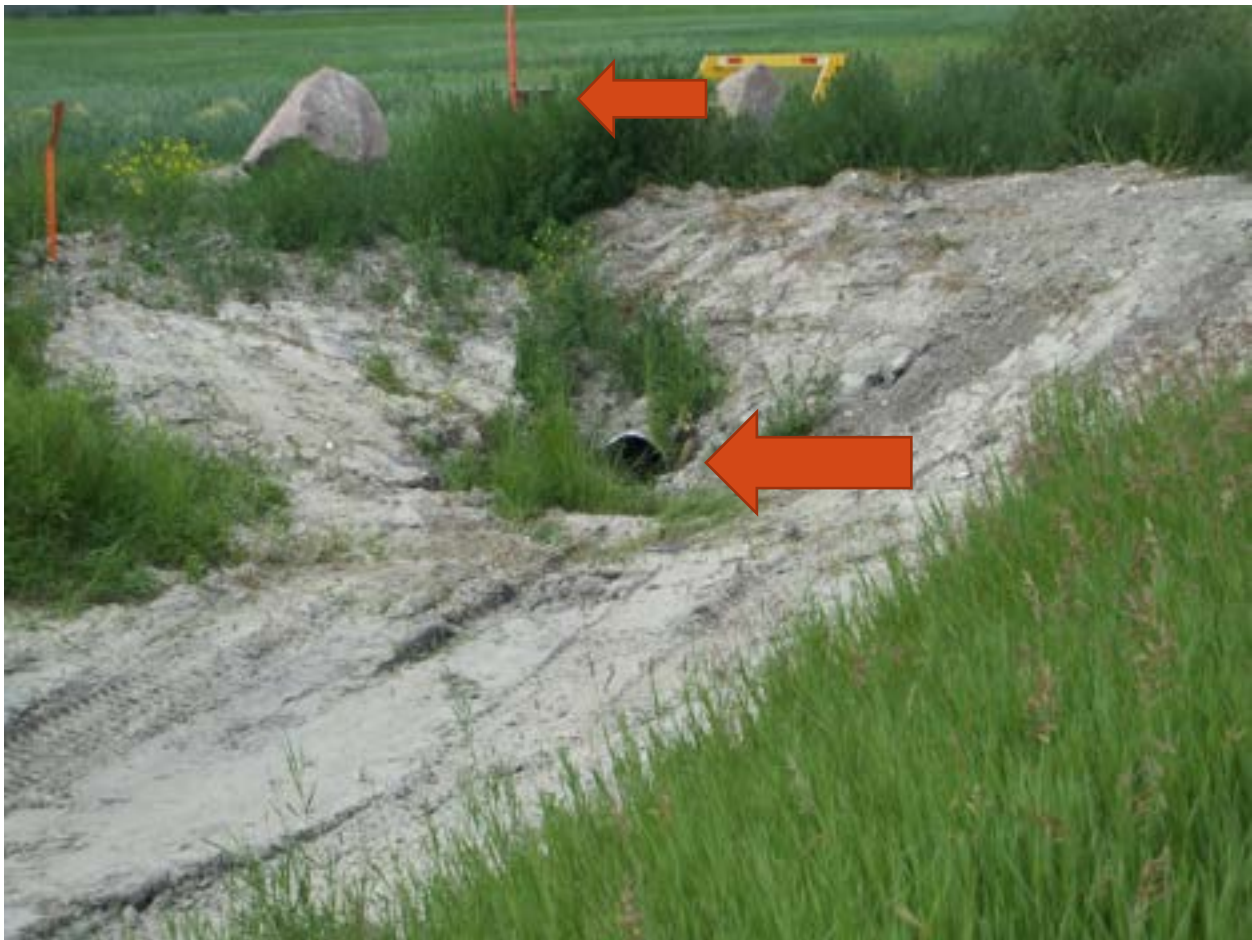
Figure 9. New, longer culvert (bottom arrow) installed in widened field access driveway across ditch at West well. Note the ludicrously tiny culvert diameter. Wellhead is at top left of centre behind weeds (top arrow).
