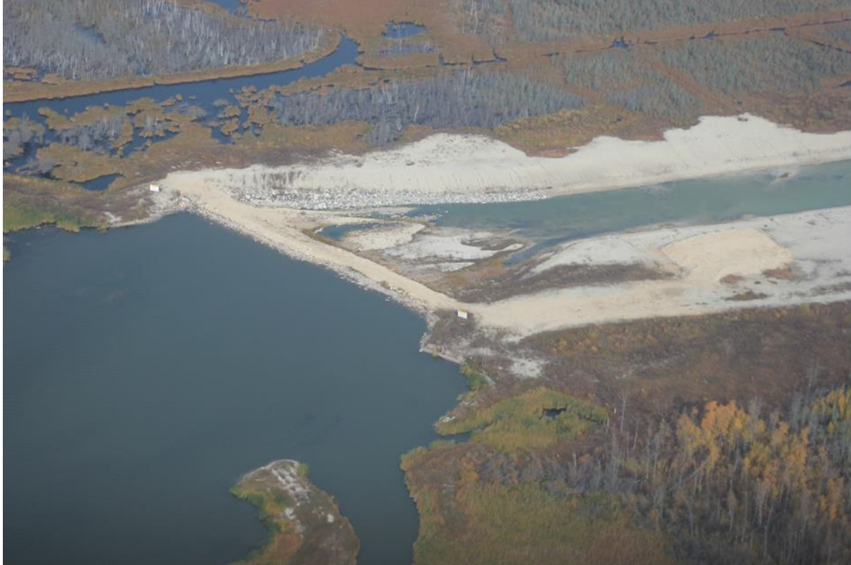
Photograph 1-2. Lake St. Martin Emergency Outlet Channel Clay and Aggregate Berm
