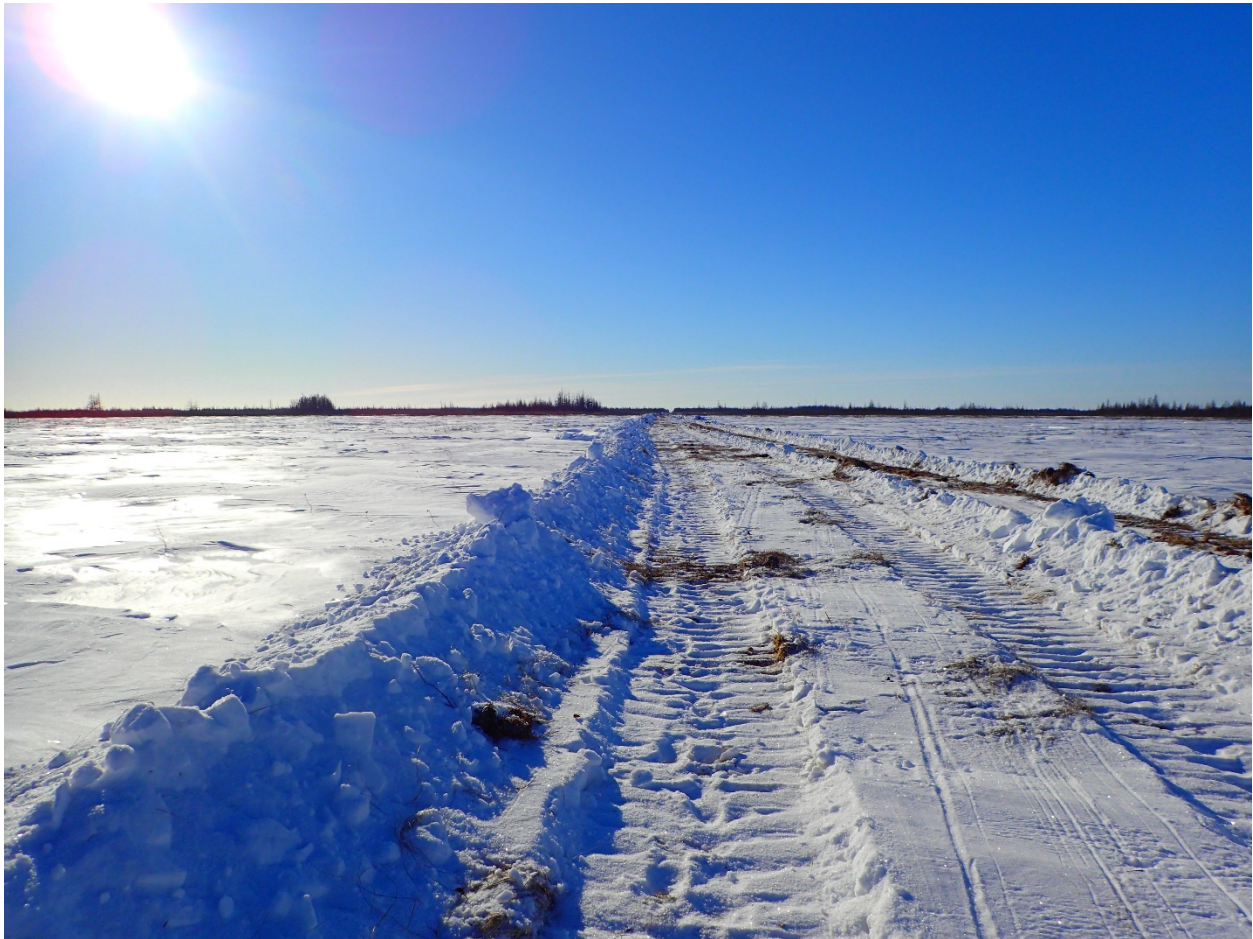
Photograph 2-1. Picture of the Winter Road
