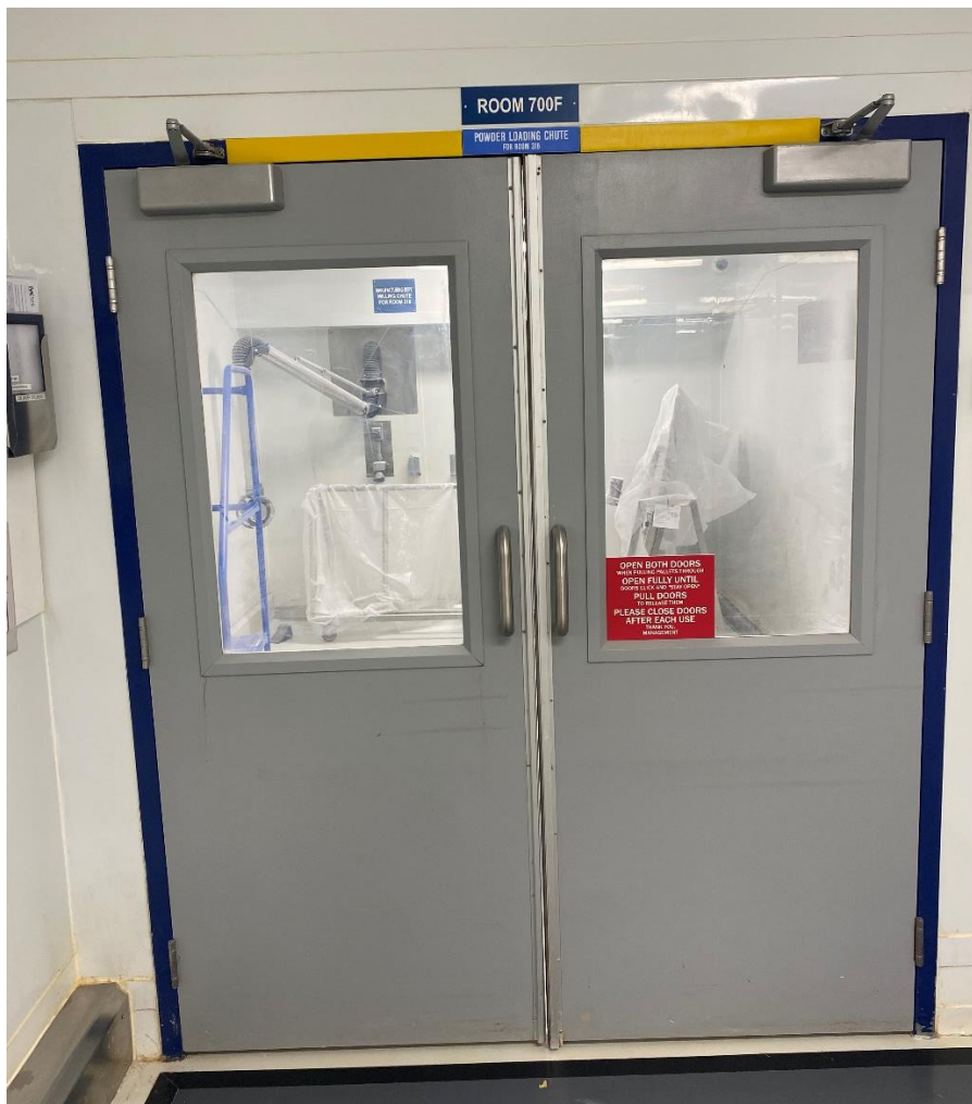
Figure 1: Room 700F (Powder Loading Chute)
