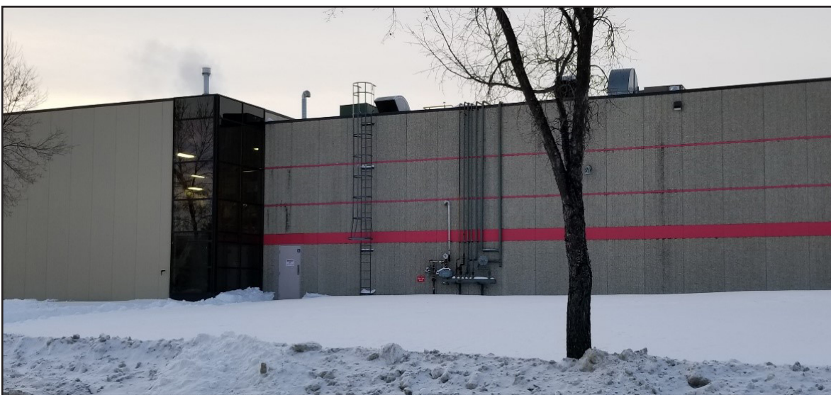
Photo B-2: Vita Health building structure from Paquin Road, facing south.
