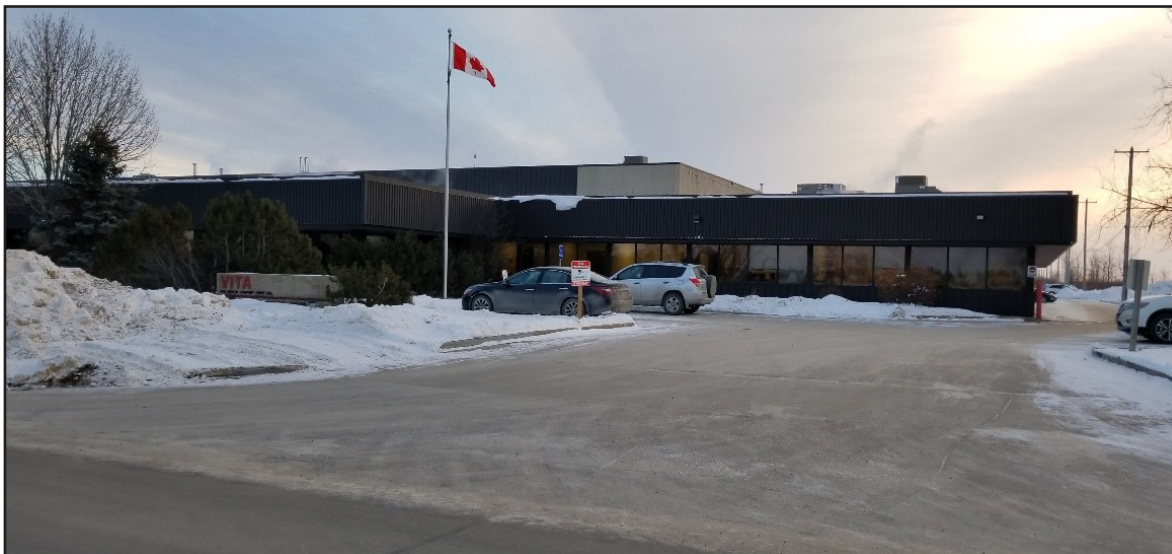
Photo B-1: Vita Health manufacturing facility at 150 Beghin Avenue, facing east.
