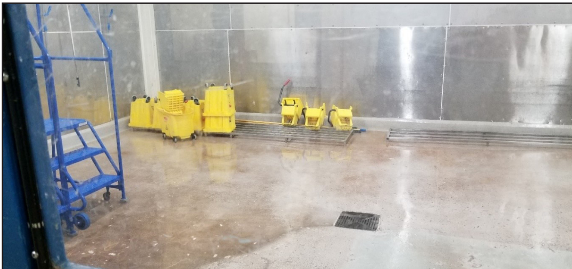
Photo B-11: Floor drains in the equipment cleaning rooms of the manufacturing area.
