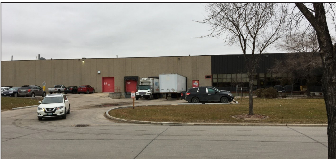
Photo B-19: Shipping area on the west side of the facility, showing the 4 bays and parking areas.
