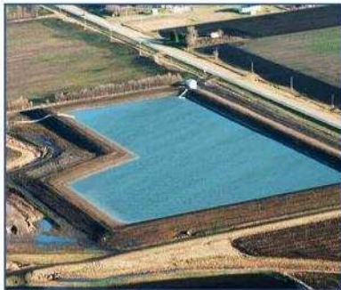
Figure 1. Water storage reservoir near Gnadenthal, MB (JKW Construction).
