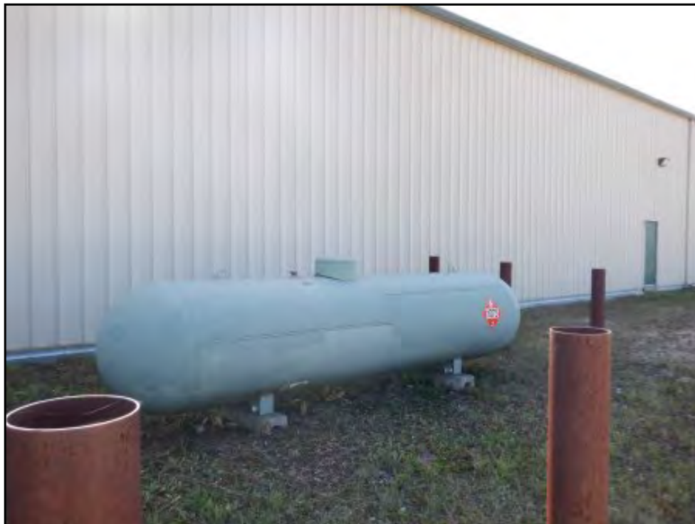
View of propane AST located on the northern side of the arena.
