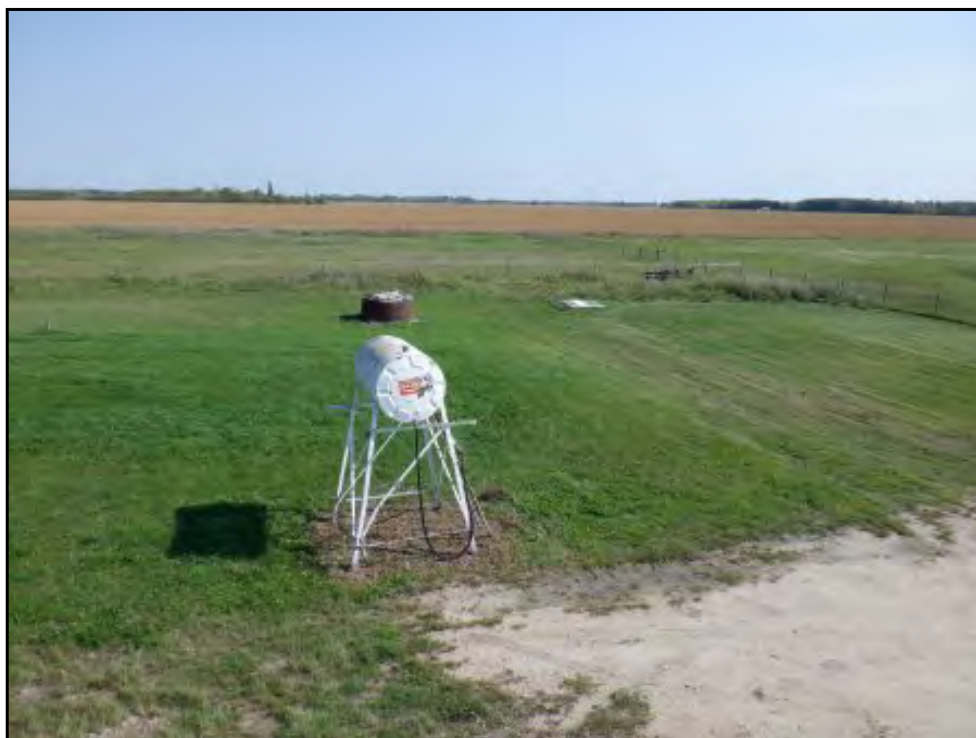
View of AST on the east side of the house. Note the stressed vegetation under the tank (1/2).
