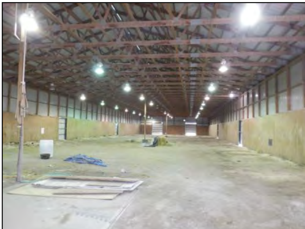
View inside south half of barn.
