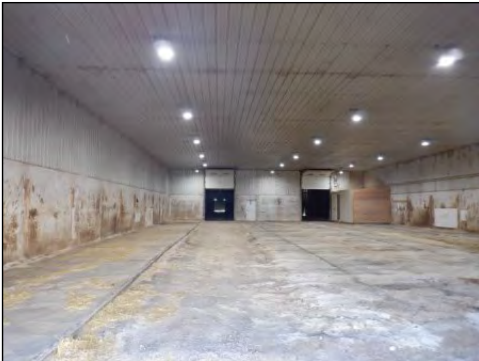
View inside north half of barn.
