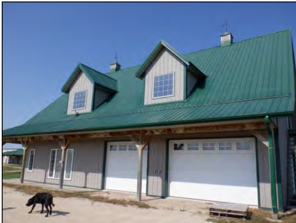
View of the south exterior of the house.
