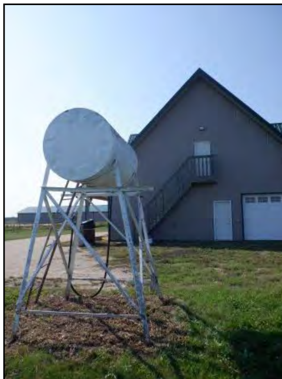
View of AST on the east side of the house. Note the stressed vegetation under the tank (/2).
