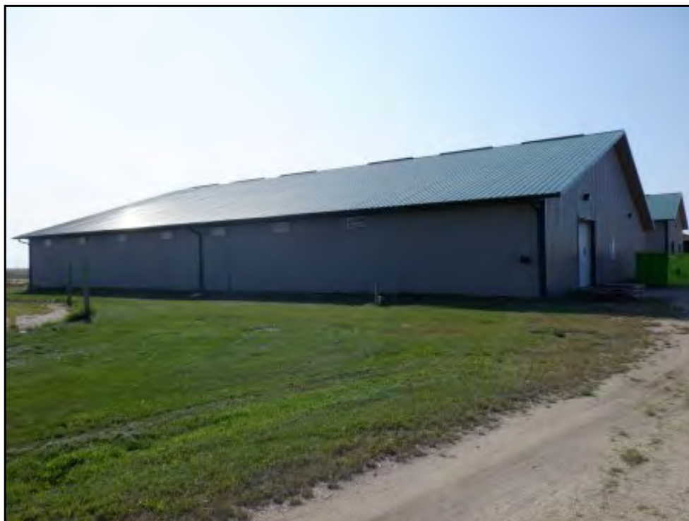
View of east/north sides of the stables.
