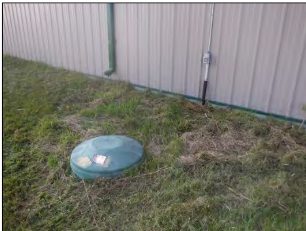
View of septic tank on east side of the stables.
