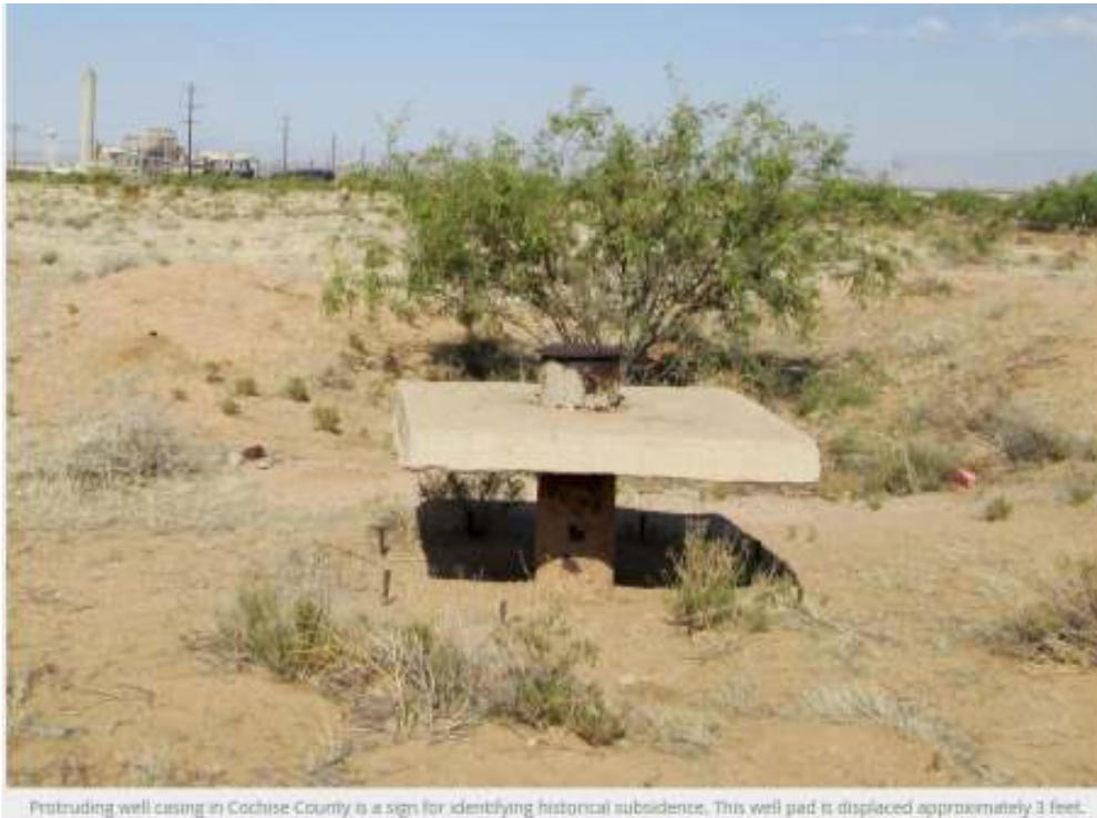
Protruding well casing in Cochise County is a sign for identifying historical subsidence. This well pad is displaced approximately 3 feet.
