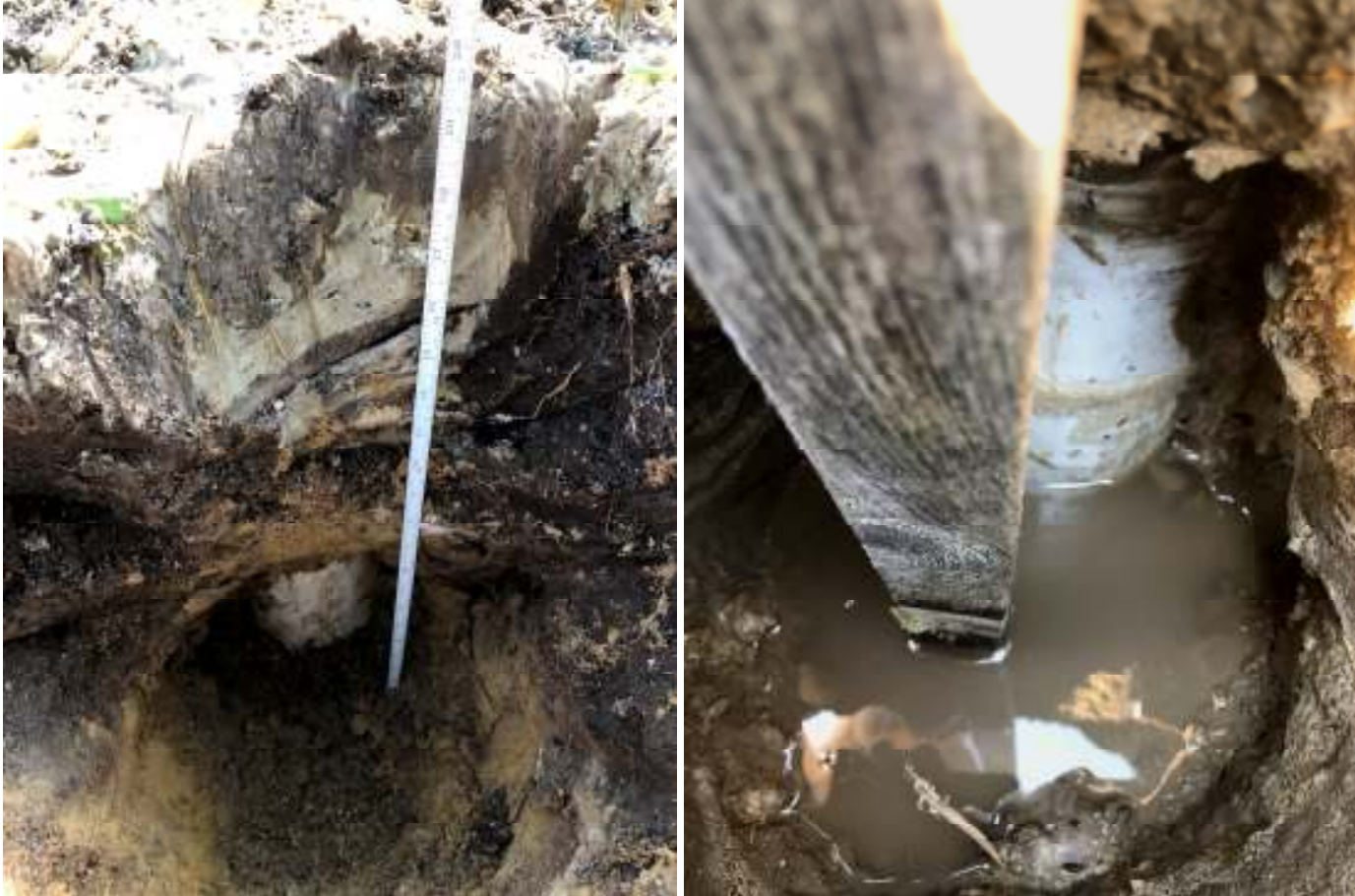
Figures 21 a and b Showing inspection by Dennis LeNeveu and Tangi Bell of the sealing of an abandoned CanWhite borehole near Ross Manitoba.
