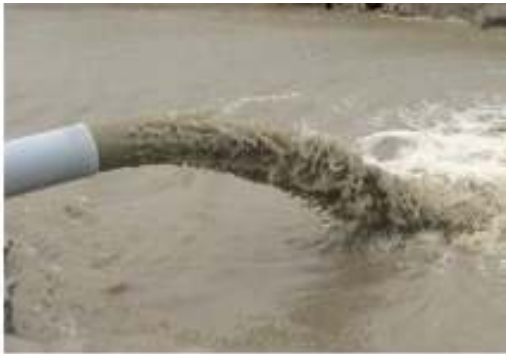
Figure 2. Beach sand slurry discharge containing 15% solids, 85% water in Japan.
