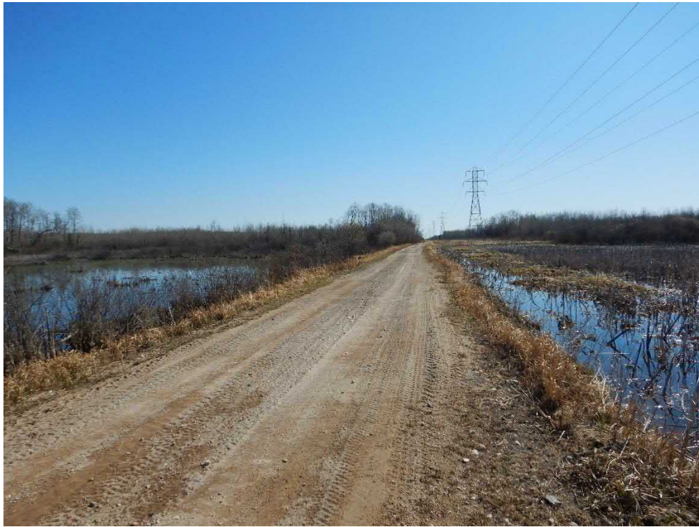
Figure 6. Existing Access Road leading to PSA. Note transmission line and marshland.
