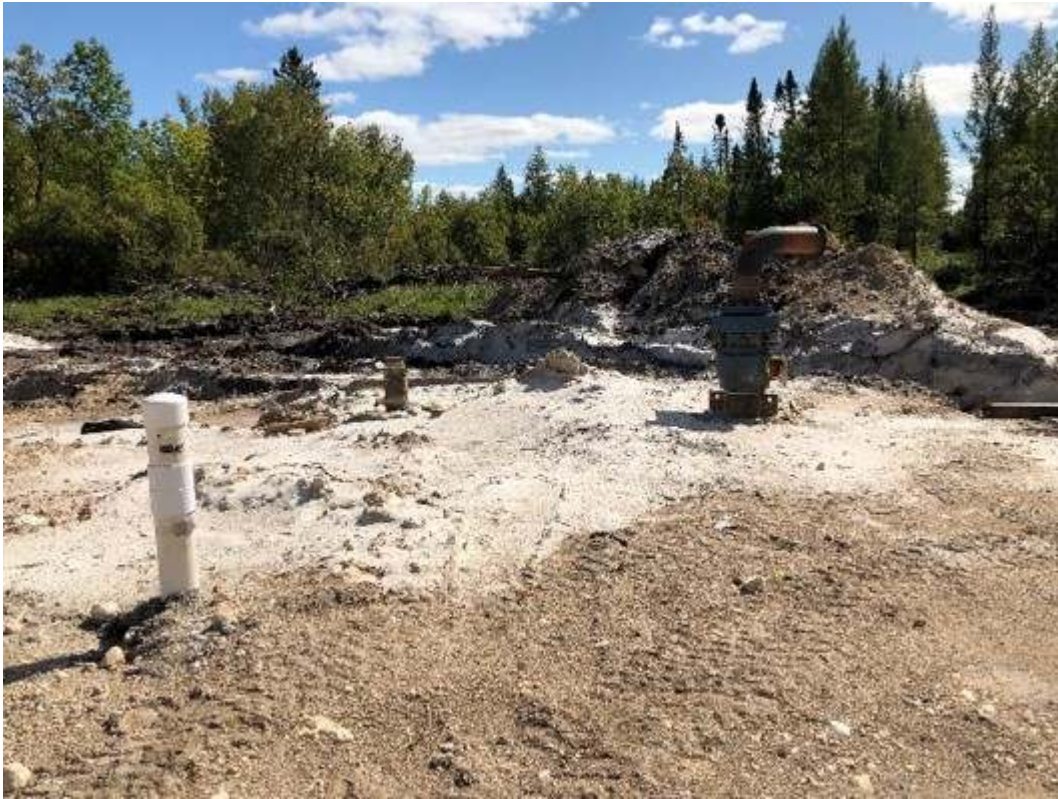
Figure 17. Unsealed CanWhite boreholes near Vivian spring, 2020.
