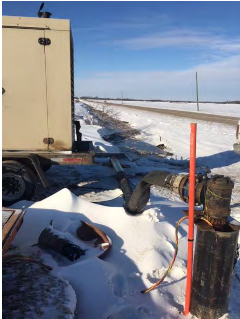
Figure 23 – West Production Well and Discharge Set Up
