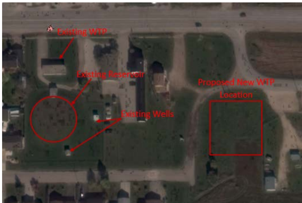
FIGURE 2.1 – LOCATION OF WTP (GOOGLE EARTH, 2018)
