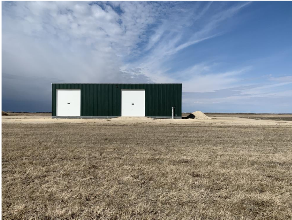
PHOTOGRAPH 1: Overview of Site buildings, facing west.
