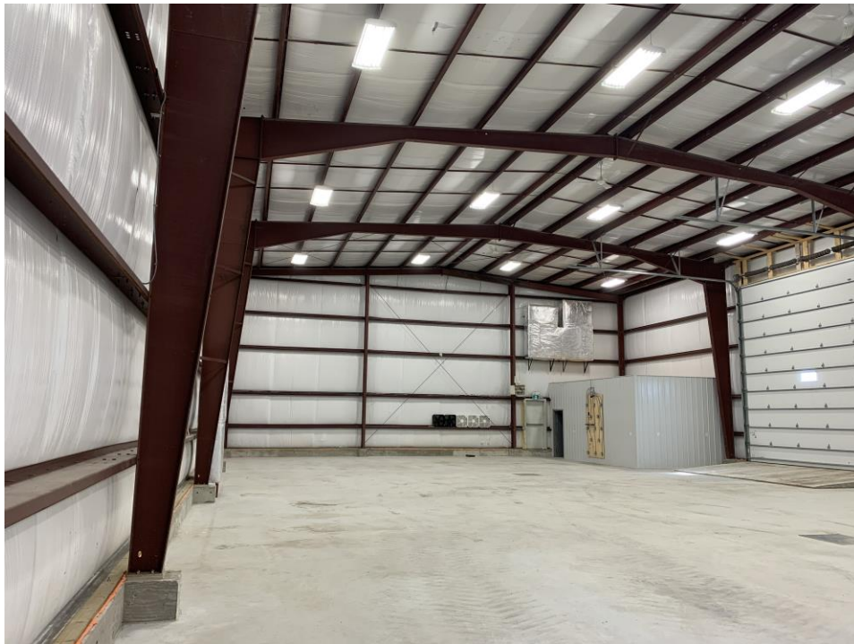
PHOTOGRAPH 2: Interior of Site building.
