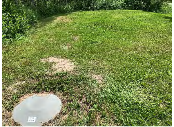
1.8 Fiberglass Wastewater Holding Tank Access Hatch on Septic Field
