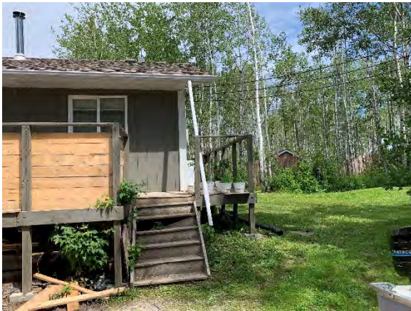
1.9 Public Washroom/Shower Building and Adjacent Septic Field
