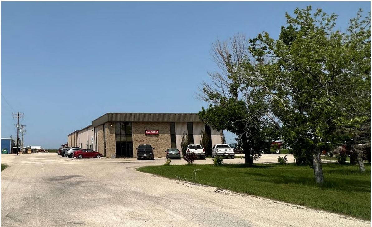
Photo 2: General view of office/ warehouse building. View looking north. (Tetra Tech, June 2023)
