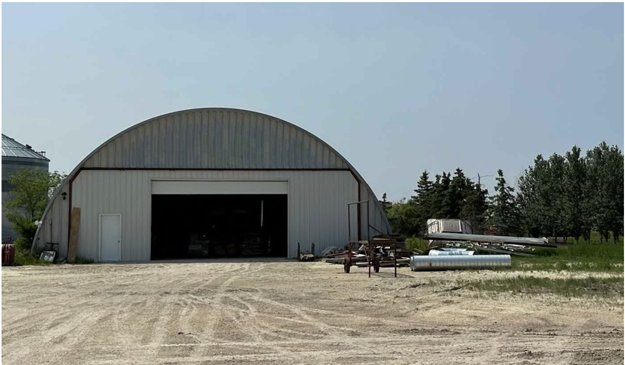
Photo 4: General view of Quonset storage building in northwest corner of site. View looking west. (Tetra Tech, June 2023)
