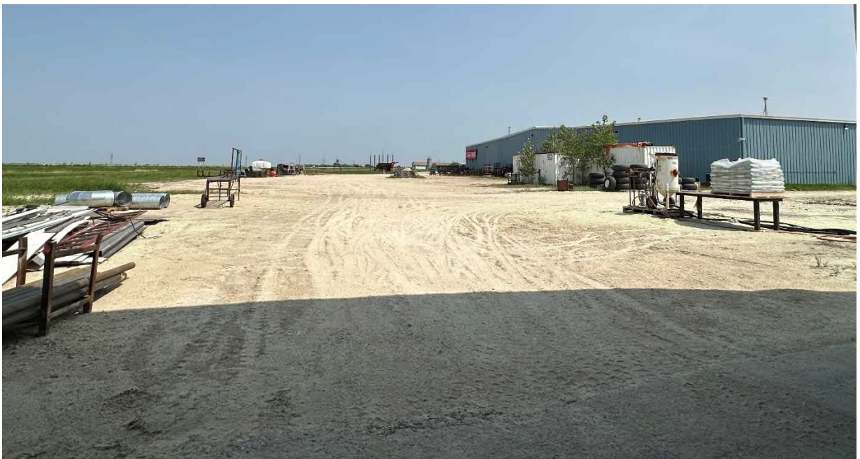
Photo 6: General view of outdoor storage area on north edge of site. View looking east. (Tetra Tech, June 2023)
