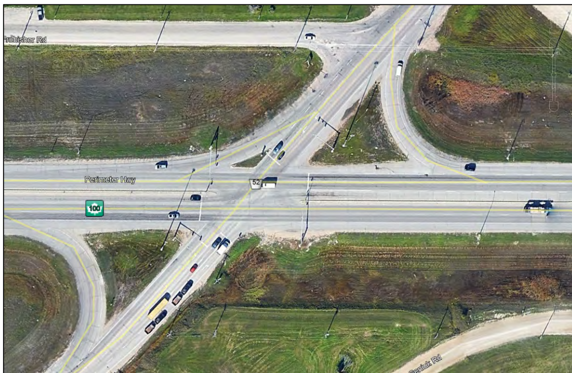
Figure 2. Existing Intersection Configuration
