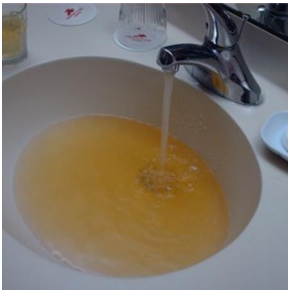
Figure 12. Untreated iron-containing well water that has been exposed to oxygen prior to emerging at the tap. Source: https://www.idahowatersolutions.com/water-problems-solutions/iron-in-water-is-it-harmful
