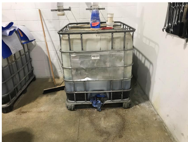
Photo 6: Sulphate Wastewater Tote – wastewater is piped into the tote via overhead piping. Totes are emptied by Miller Environmental approximately twice a year as limited amount of chromic wastewater is generated due to the water being recycled and reused during operations.
