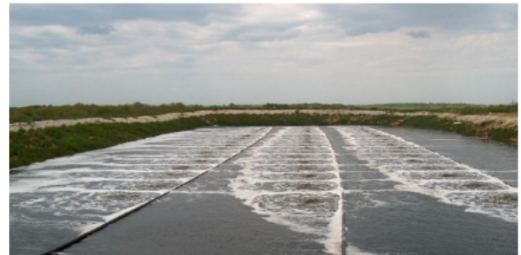
Figure 6.2: Aerated Lagoon System (Source: NEXOM)
