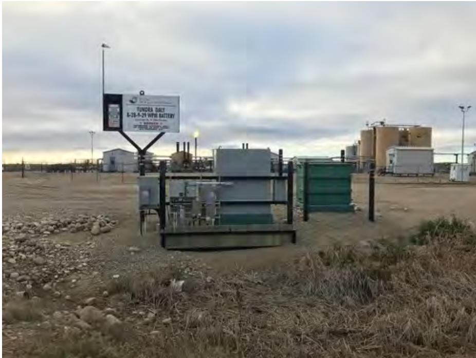
19. Looking west at Tundra Daly 08-28-009-29 W1M battery site.
