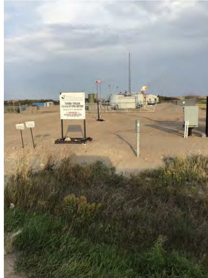
62. Looking east at Tundra Sinclair Battery 13-14-008-29 W1M battery site.
