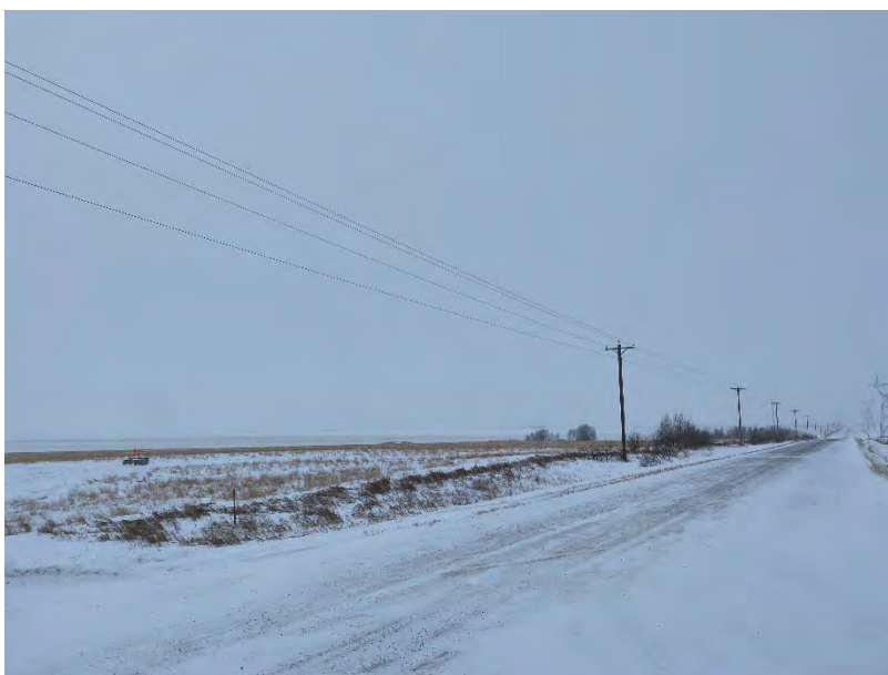
Photo 2. Start of pipeline facing northwest at section C102.
