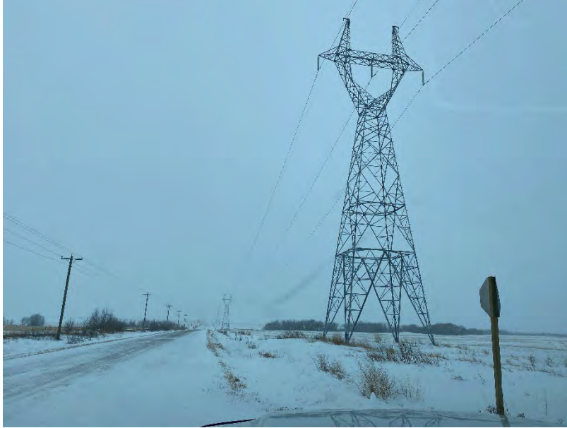
Photo 3. Start of pipeline facing west at section C102.
