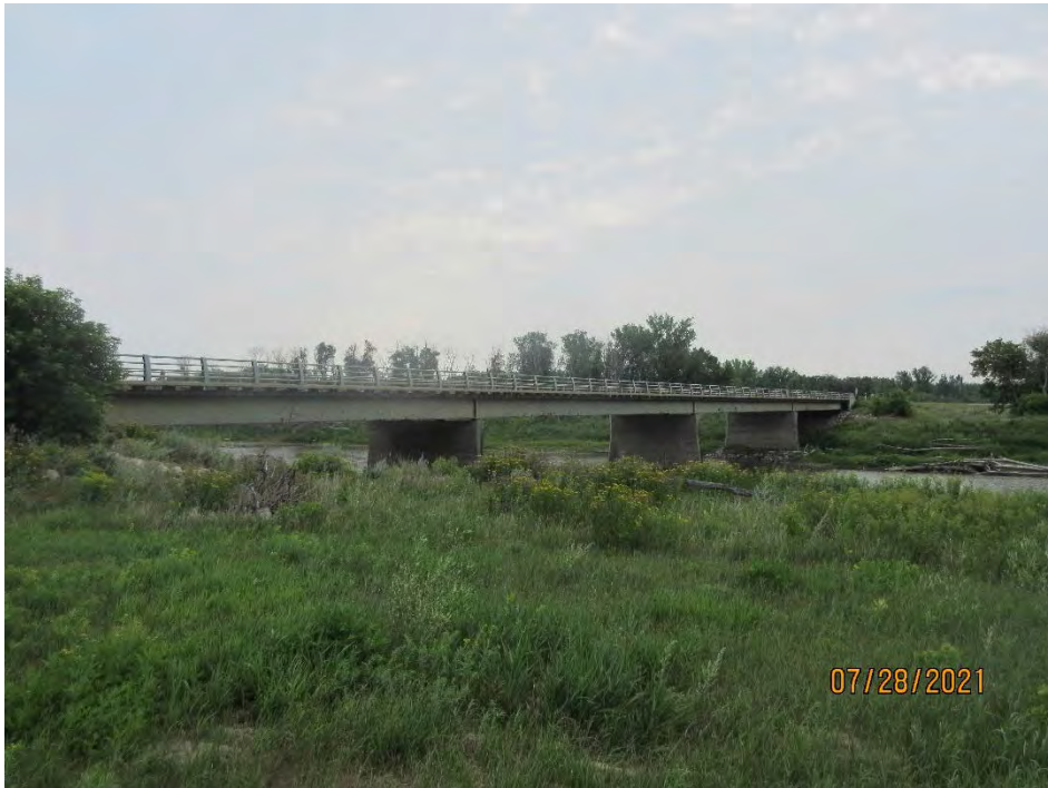
Photo 6: Looking at the upstream side of the Assiniboine River bridge from the north bank (2021-07-28)
