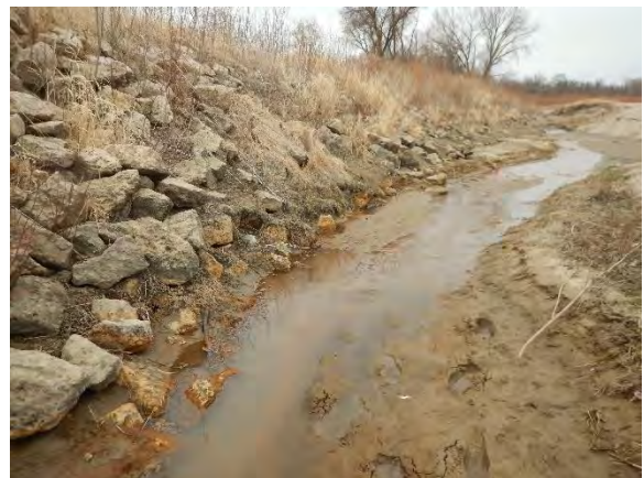
upstream view from T4, 100 m downstream of crossing
