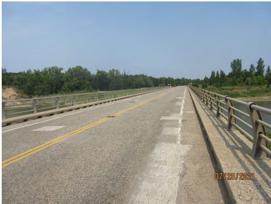
Photo 2: Looking North along PTH 5 across the Assiniboine River bridge (2021-07-28)
