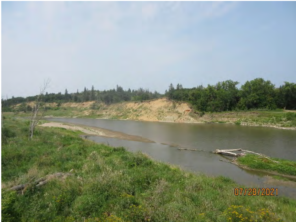
Photo 8: Looking upstream from the south bank of the Assiniboine River bridge (2021-07-28)
