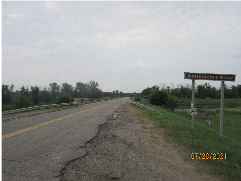
Photo 1: Looking south along PTH 5 at approach to Assiniboine River bridge (2021-07-28)
