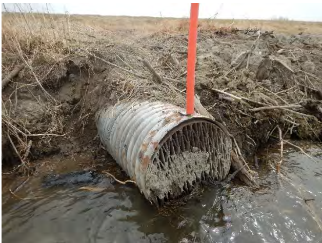
View of the culvert inlet showing the screen cover
