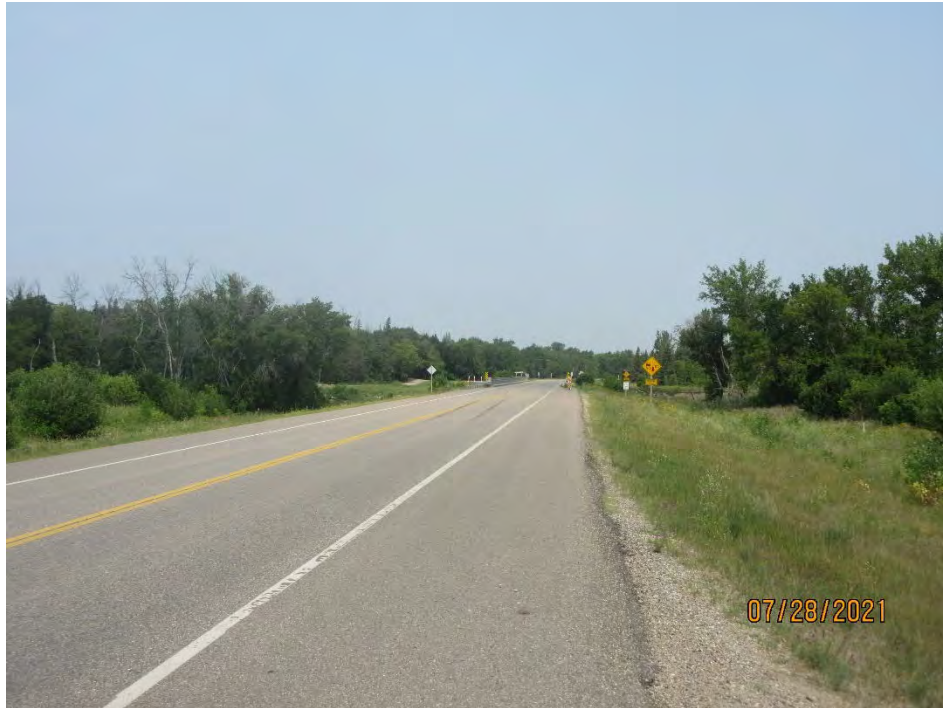
Photo 3: Looking north along PTH 5 ROW at approach to Assiniboine River bridge (2021-07-28)
