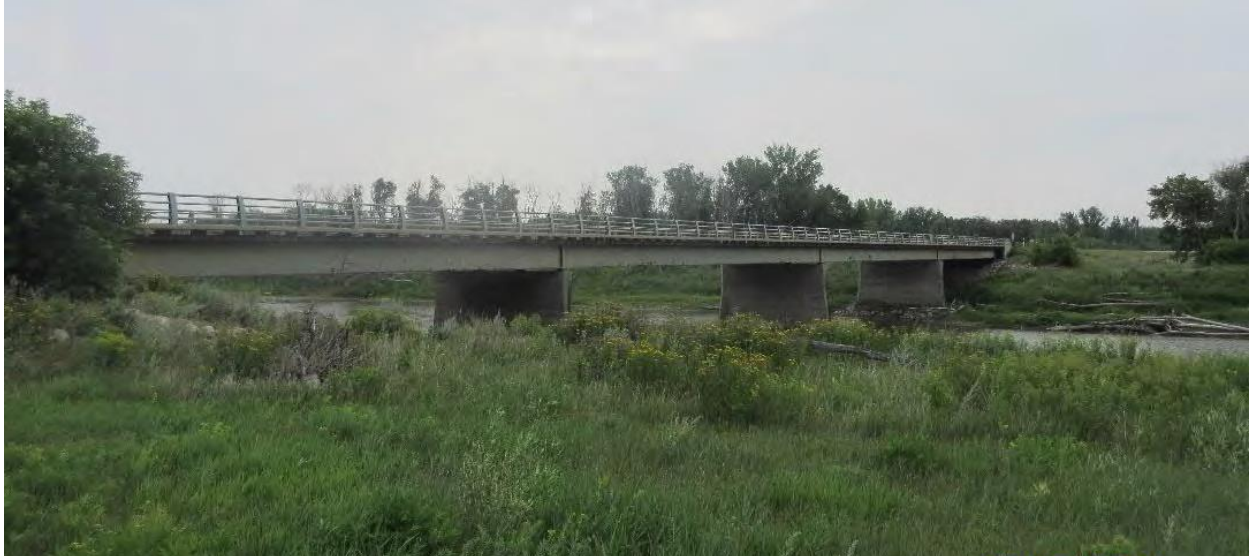
Figure 2. Existing PTH 5 bridge over the Assiniboine River (photo: KGS 2021).
