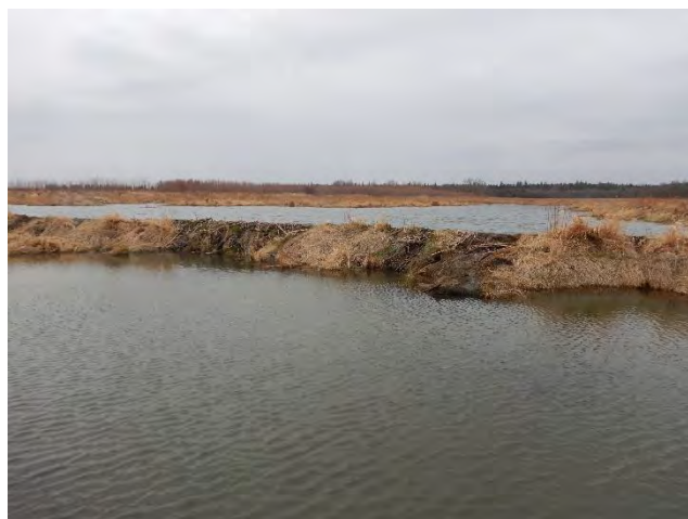
Large beaver dam downstream of culvert crossing
