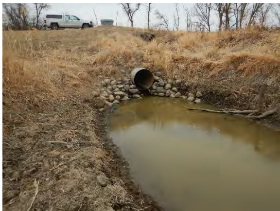
Upstream view from T3, 5 m downstream of crossing
