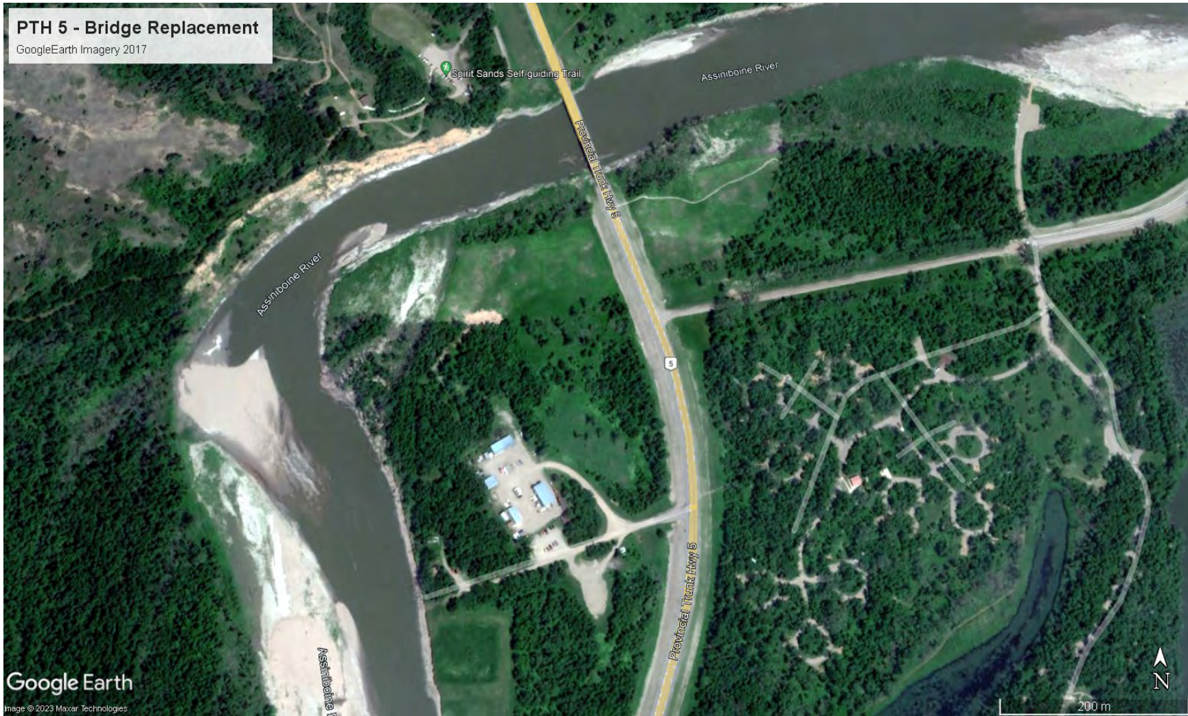
Figure 3. GoogleEarth Image from 2017 of Site and Proposed Relief Bench showing erosion and tree clearing completed for the relief plug which was not constructed
