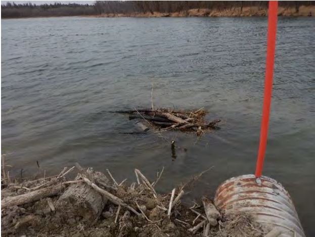
Upstream view from the culvert crossing
