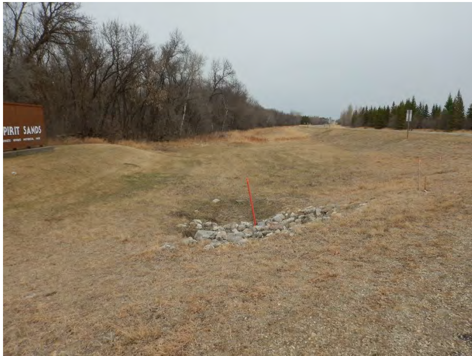
Upstream view from the culvert crossing
