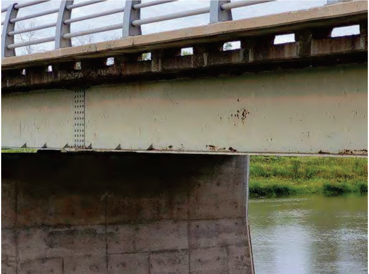
Cliff swallow nests on the underside of the existing bridge structure.
