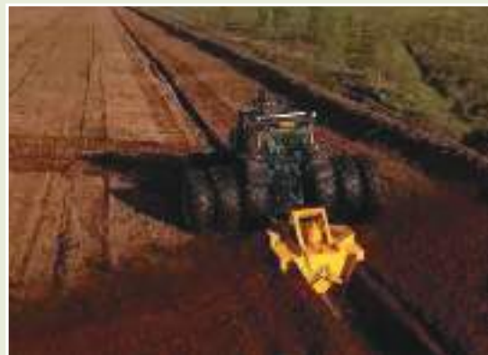
Field Drain Construction with Typical Profile of 1.5m x 1.5m at ~33m Intervals
