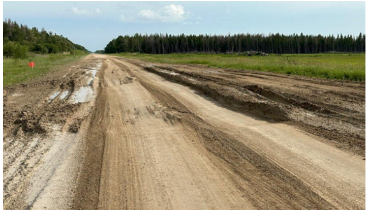
Figure 3. Provincial Road 234 reduced to a single track with foot-deep ruts, July 3 2024 [12].
