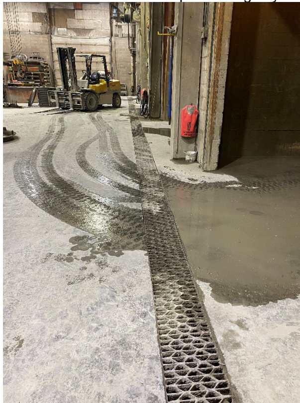
Photo 12. Wet catch channel outside cutting bay door.
