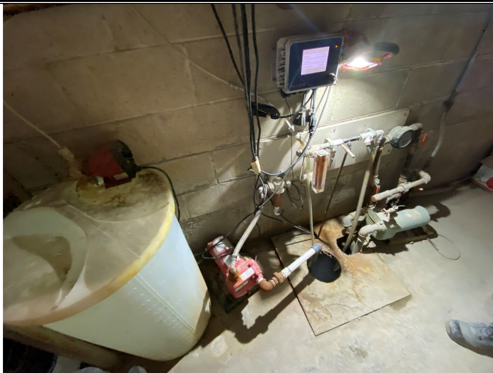
Photo 13. Hydrochloric slurry treatment system over holding tank.
