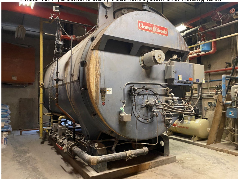
Photo 14. On-Site natural gas boiler.
