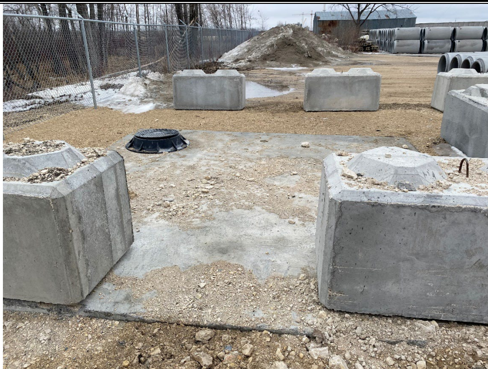
Photo 15. Process effluent holding tank with concrete block barriers.
