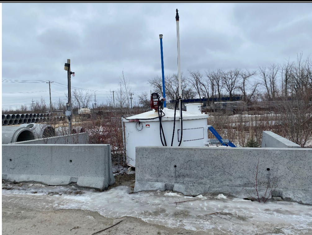
Photo 17. Diesel Fuel AST on Site.
