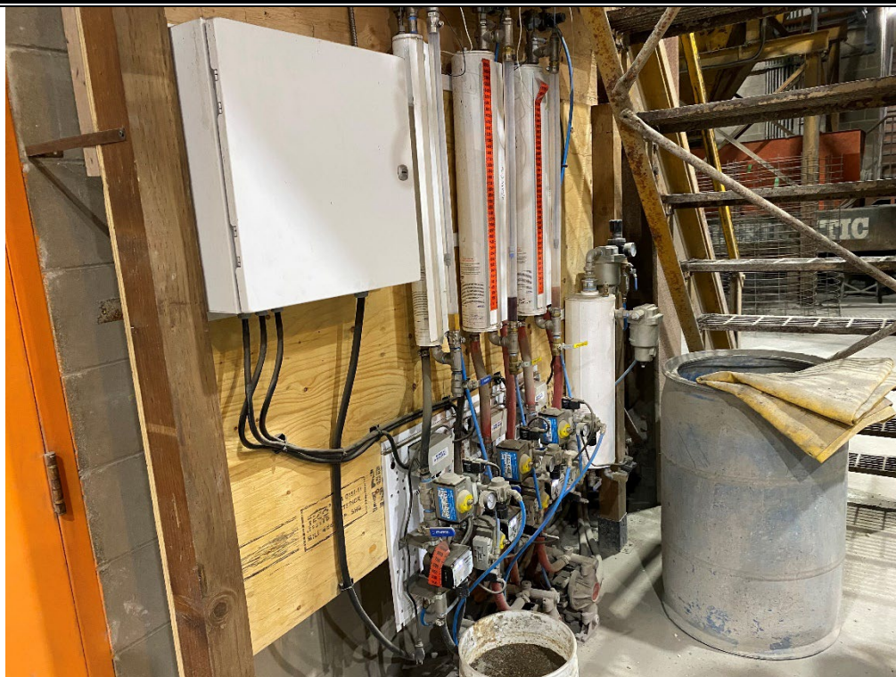
Photo 9. Additives distribution valve network.
