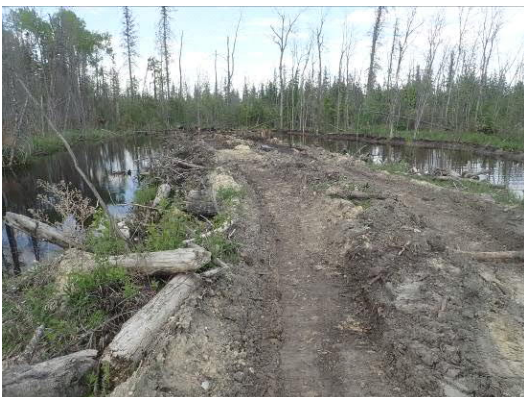
Photo 5: Existing overland discharge area at end of Evergreen 2/3 outlet ditch.
