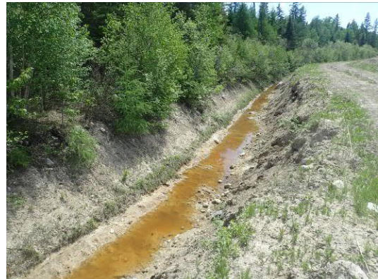
Photo 4: Existing outlet ditch for Evergreen 2/3.
