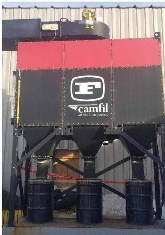
*Figure 3 – Laser dust collector/air purifier*
