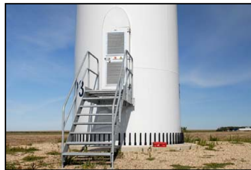
Image 13 – Tubular Monopole Tower
