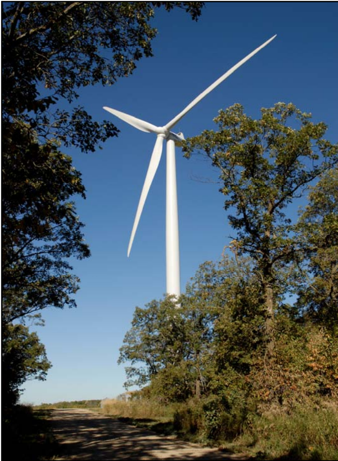
Image 10 – Height above trees to capture steady wind
