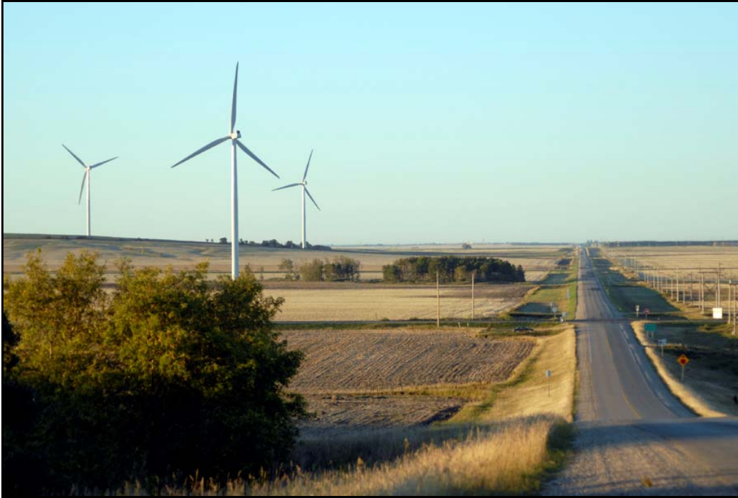
Image 2 - St. Leon Wind Farm
