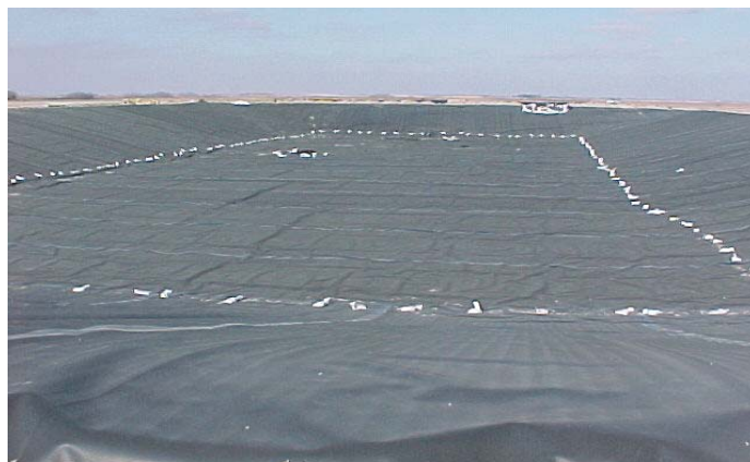
Plastic liner used to line an earthen manure storage structure
