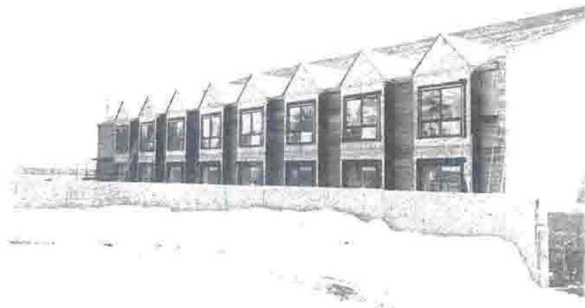
Photo 24. - New Wing to Resort under Construction
