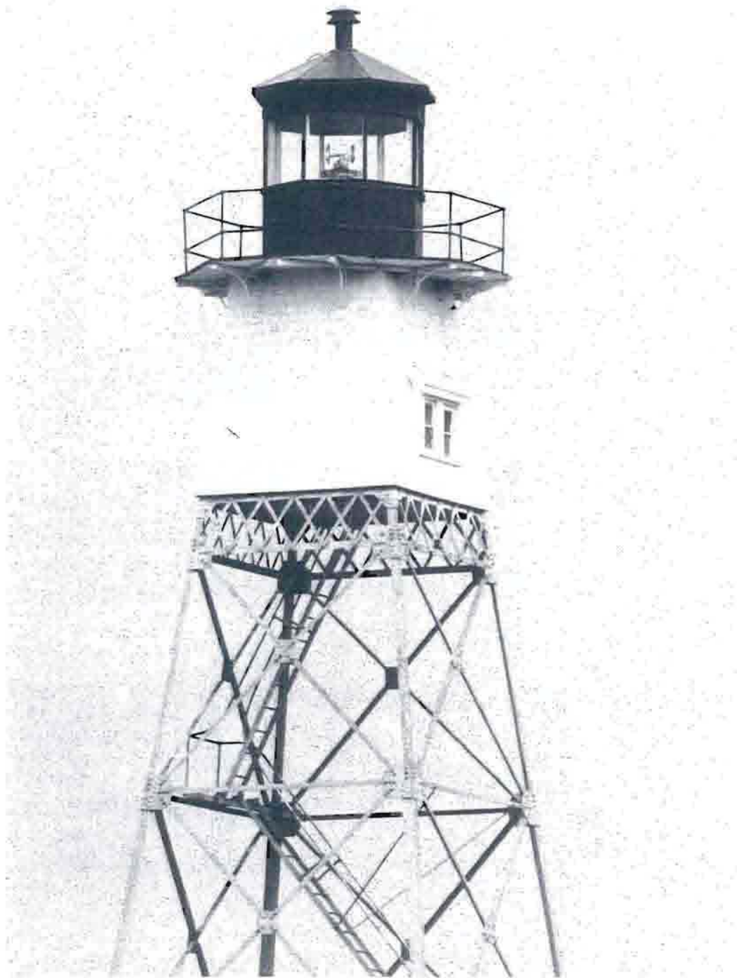
Photo 34. Beacon at Gull Harbour
