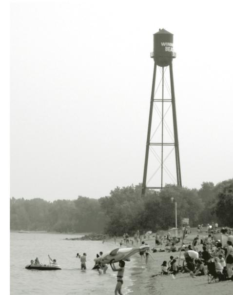
It provided pressurized water for the CPR steam locomotives and fire protection services for the resort's facilities. Out of use since the resort closed, the structure is the best example of only five surviving riveted-steel water towers in Manitoba. As in its heyday, the tower remains a prominent visual landmark in and around the beach community.
