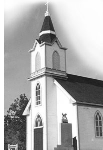
Hecla Church, restoration complete. 1973-1975
