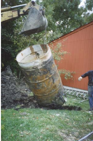
Removal of well pit cribbing
