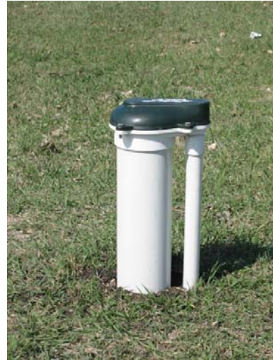
Completed well pit upgrade
