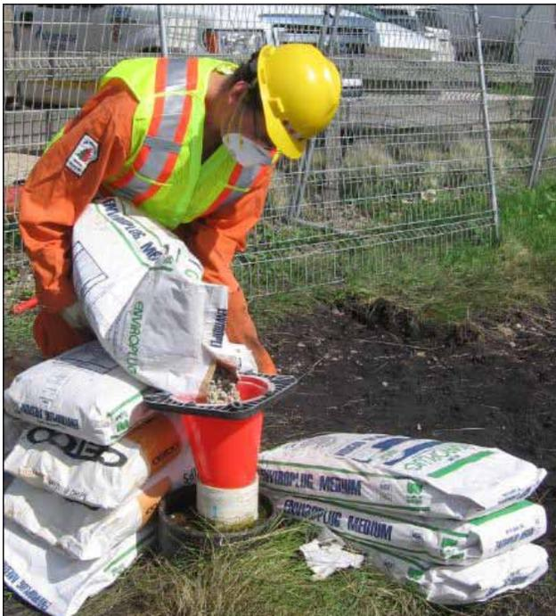
*Sealing a small diameter water well using bentonite chips.*
