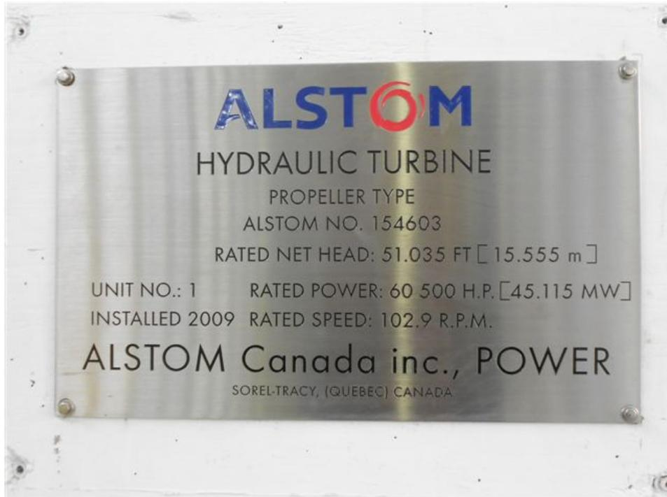
Figure 8 Unit No. 1 Nameplate Post Refurbishment, 2009
