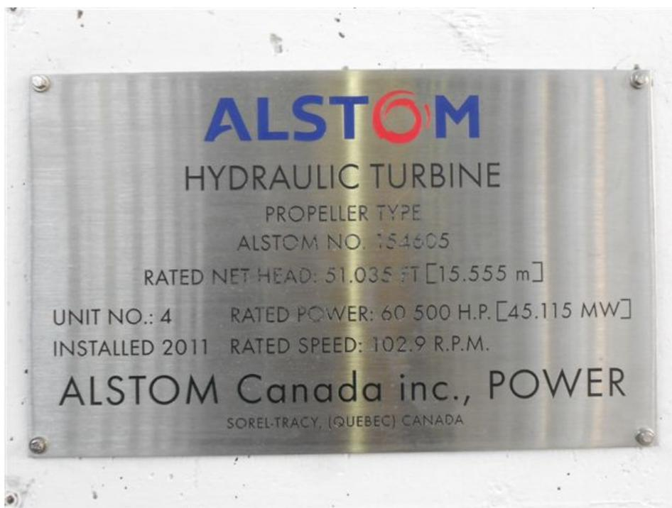
Figure 11 Unit No. 4 Nameplate Post Refurbishment, 2011
