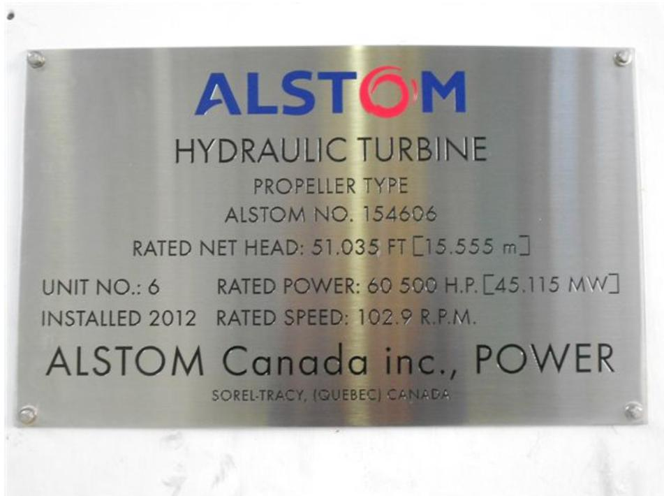
Figure 13 Unit No. 6 Nameplate Post Refurbishment, 2012
