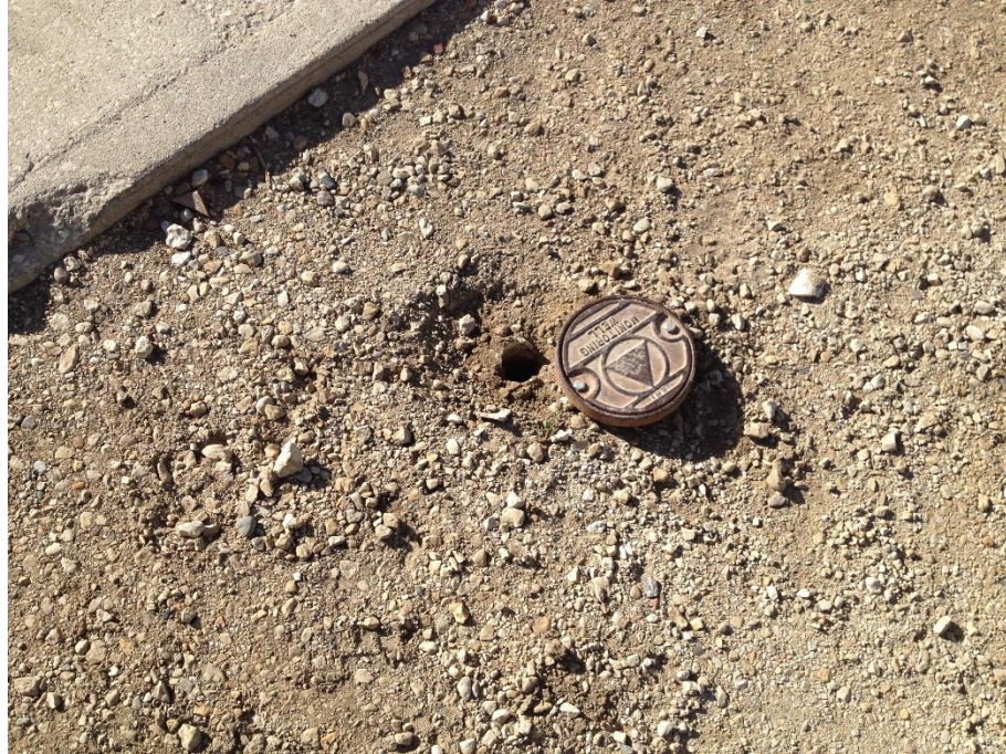
PHOTOGRAPH 5: Condition of monitoring well TH6.
