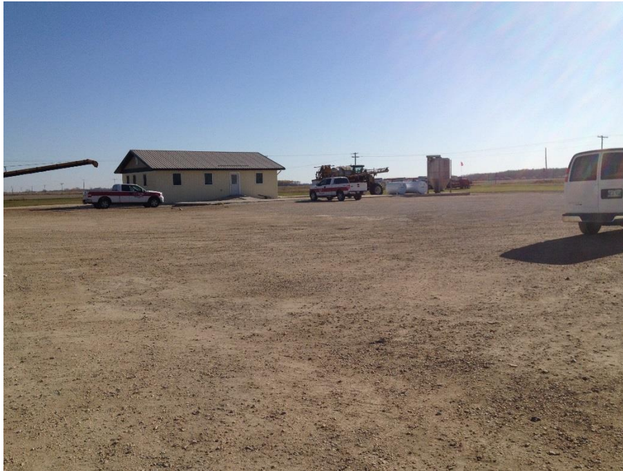
PHOTOGRAPH 3: Re-graded parking lot and new office building.
