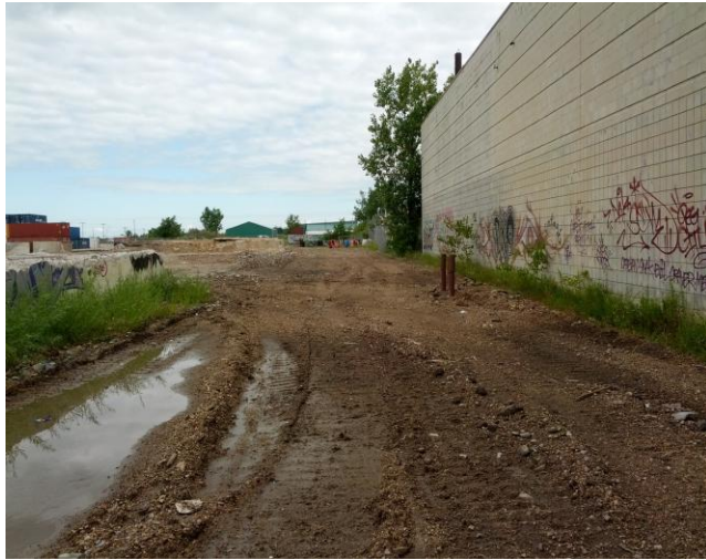
Photo 1: View looking north at 13-01, 13-02 and 13-03
