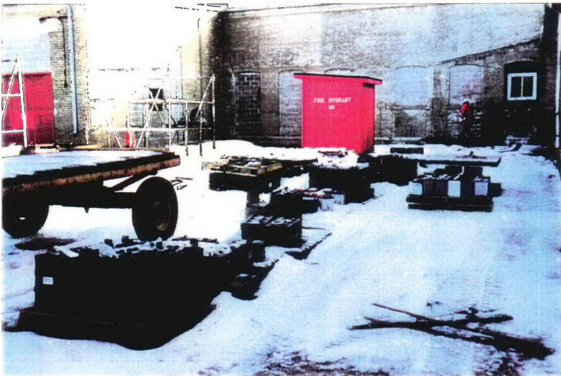
Photo 10 Battery Storage Area at Southwest Corner of West Maintenance of Way Shop
