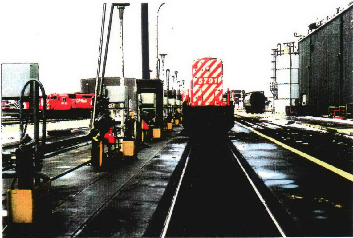
Photo 1 Winnipeg Diesel Shop Fuelling Station
