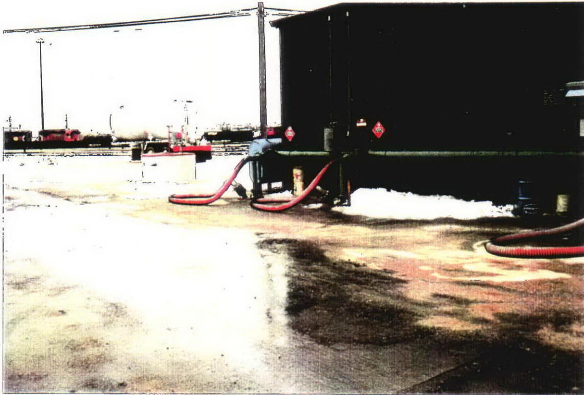
Photo 5 Truck Transfer Point at Current Fuel Storage Facility
