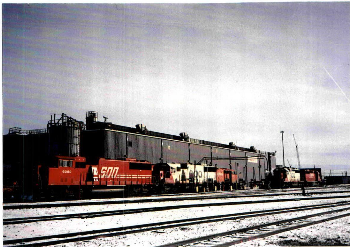
PHOTOGRAPH 1: VIEW OF ACTIVE LOCOMOTIVE FUELLING FACILITY LOOKING NORTHEAST.
