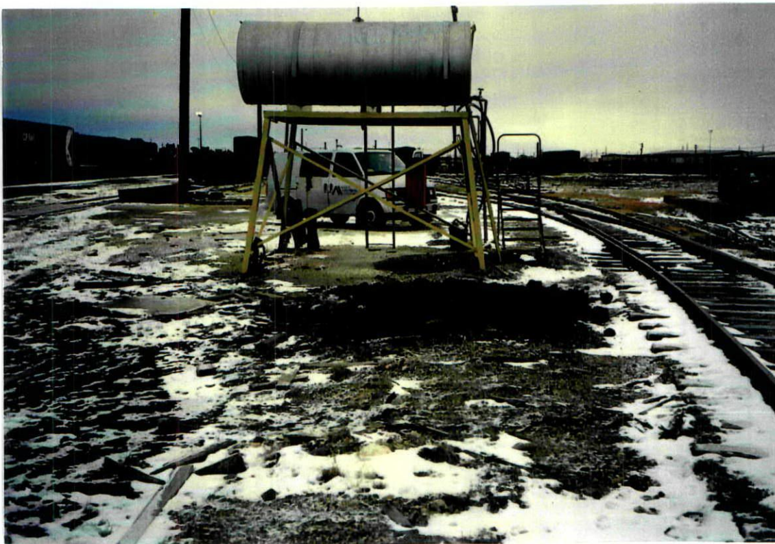
PHOTOGRAPH 4: VIEW OF ABOVE GROUND DIESEL STORAGE TANK LOOKING NORTHEAST. THIS TANK SERVICES VARIOUS RAIL MACHINERY. TEST PIT 98-1 IS LOCATED IN THE BLACK AREA IN THE FOREGROUND.
