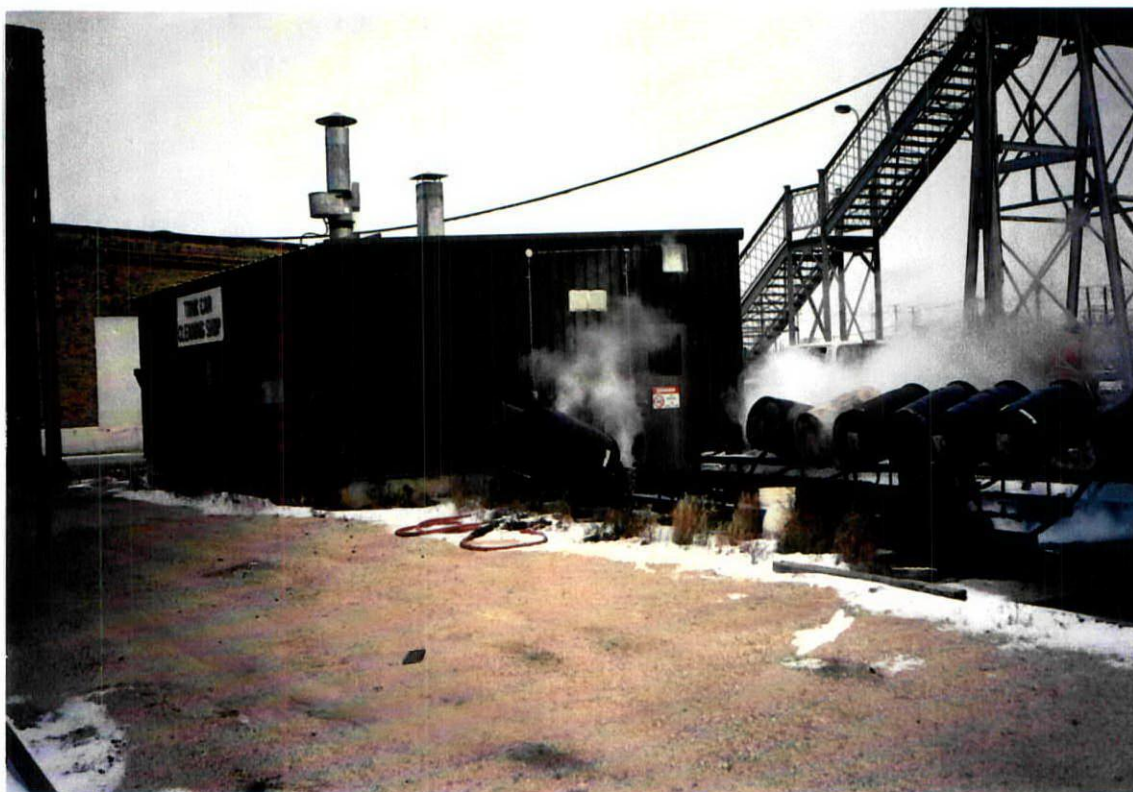
PHOTOGRAPH 6: VIEW OF FORMER TANK CAR CLEANING AREA AND THE BARREL CLEANING FACILITY LOOKING NORTHWEST.
