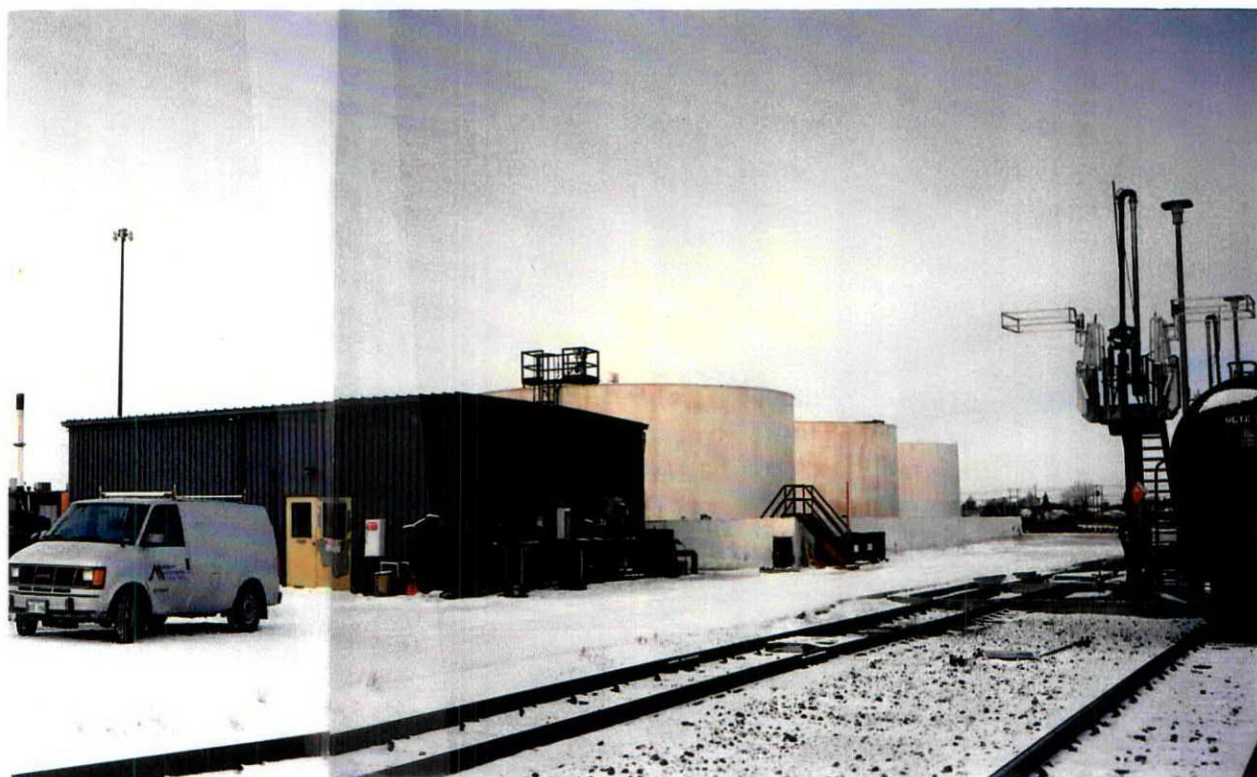
PHOTOGRAPH 2: VIEW OF ABOVE GROUND DIESEL TANKS LOOKING NORTHEAST. THESE TANKS SUPPLY DIESEL TO THE LOCOMOTIVE FUELLING FACILITY.
