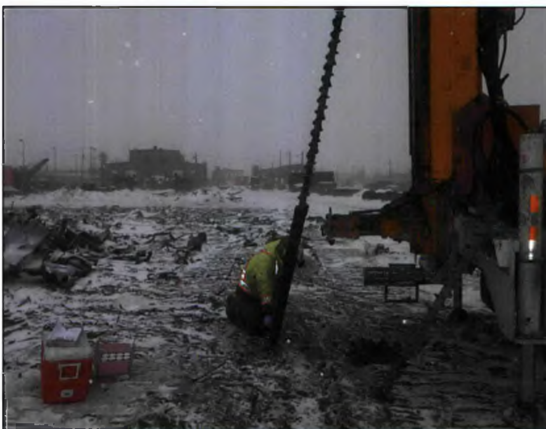
View looking east of the drill rig advancing BH08
