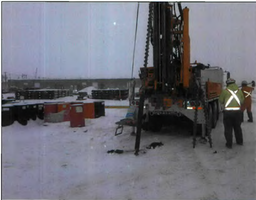
View looking west of the drill rig advancing BH02
