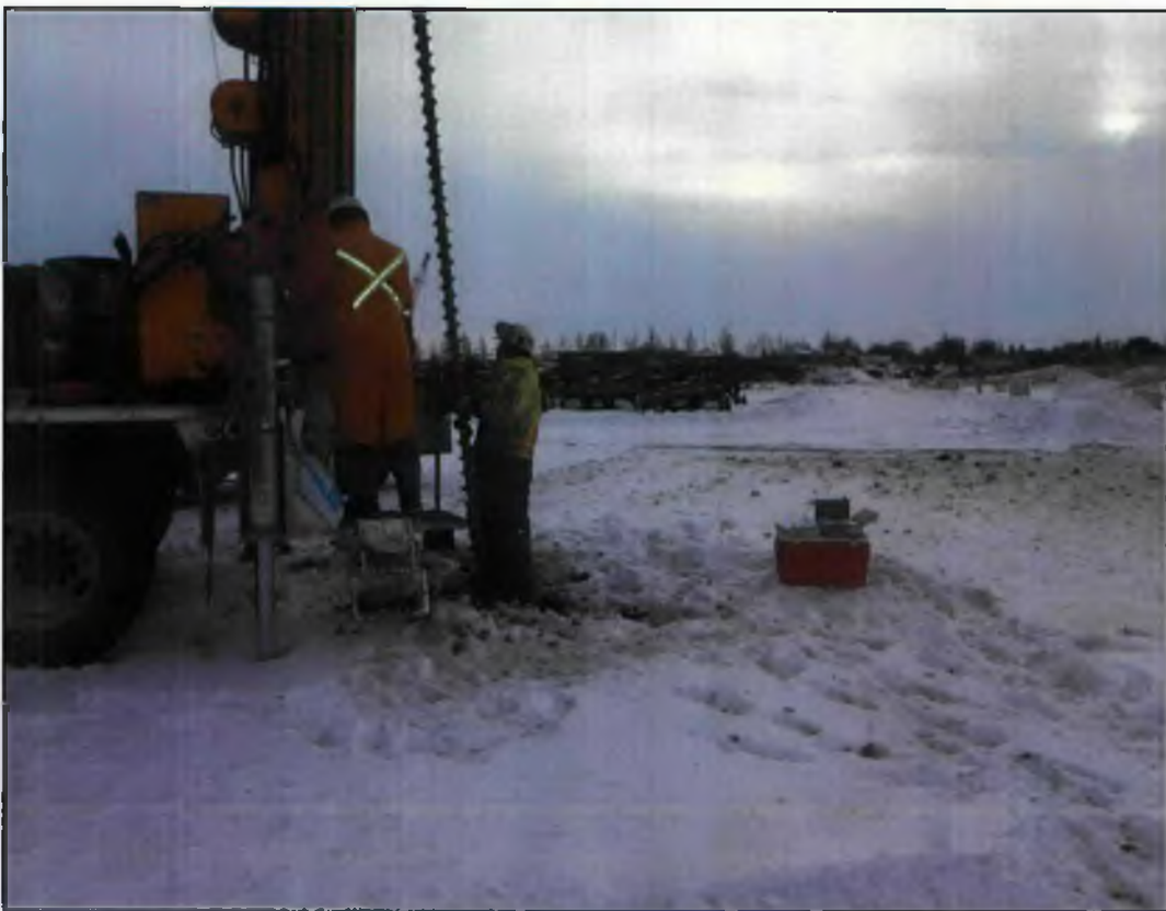
View looking southeast of the drill rig advancing BH13
