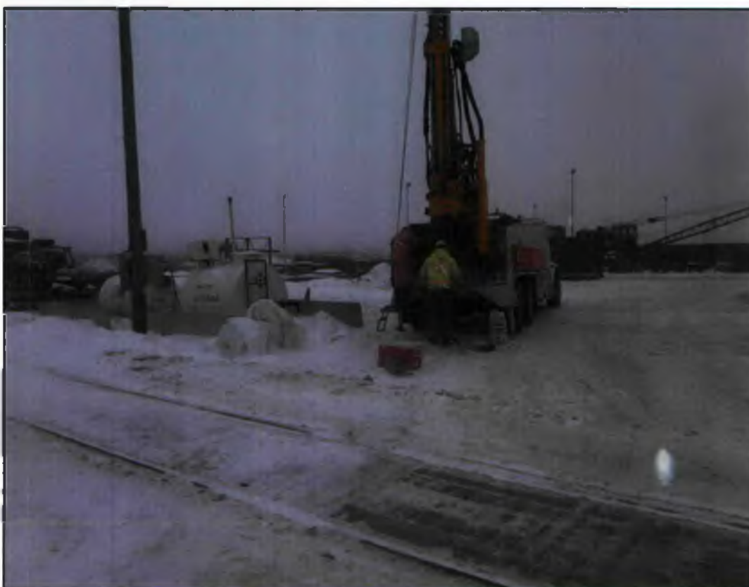
View looking northwest of the drill rig advancing BH03
