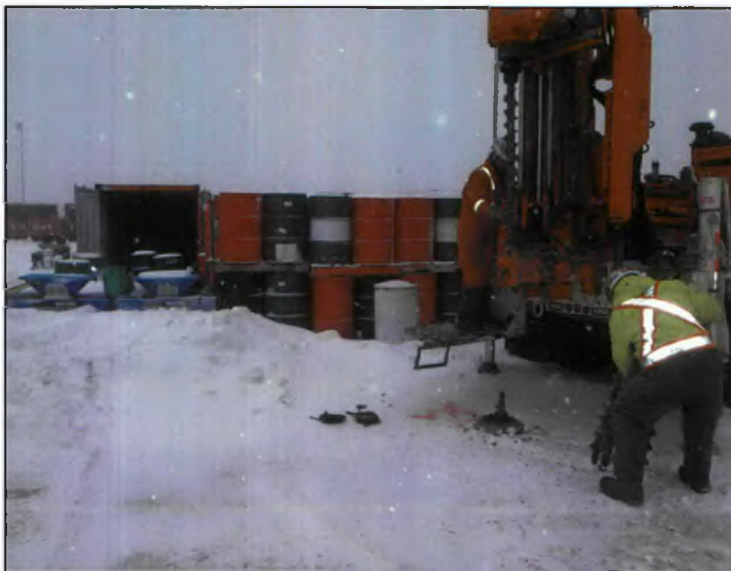
View looking south of the drill rig advancing BH01
