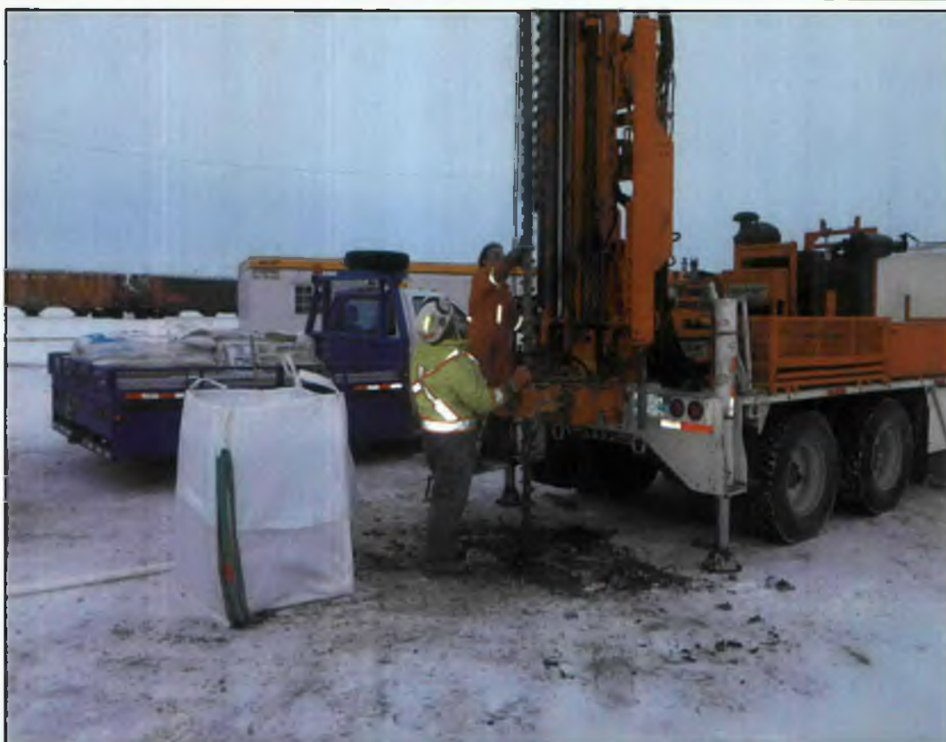
View looking west of the drill rig advancing BH07
