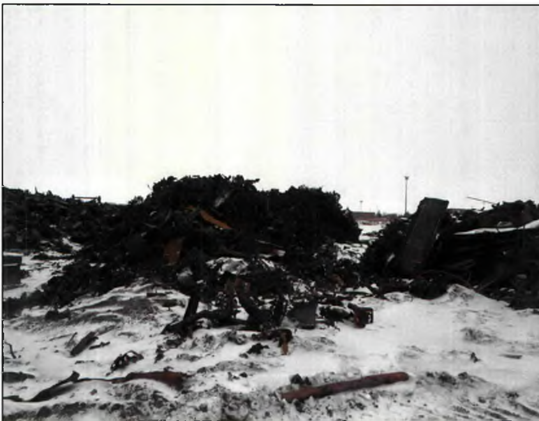
View of scrapping piles on the PR subcontractor scrapping area
