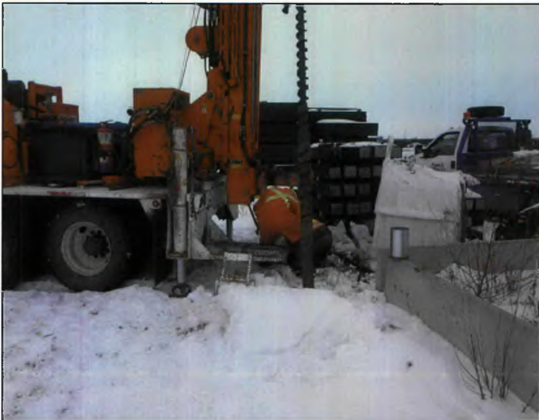
View looking east of the drill rig advancing BH05
