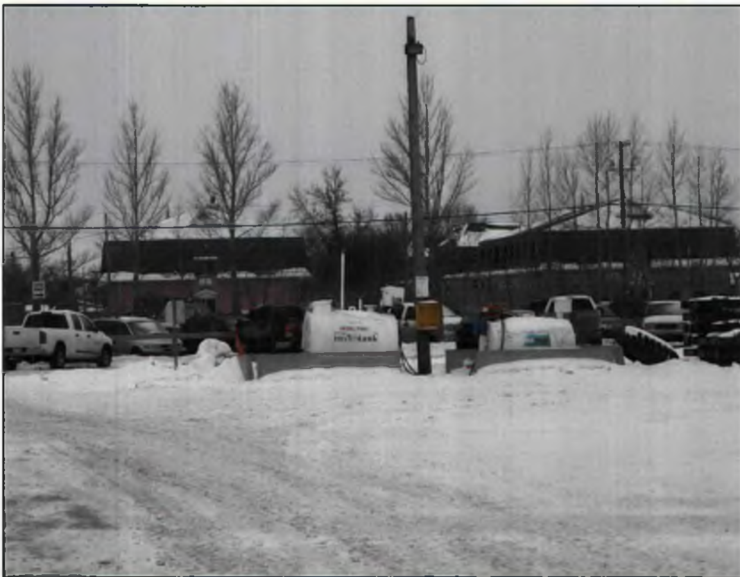
View looking south of the aboveground gasoline and diesel fuel storage tanks
