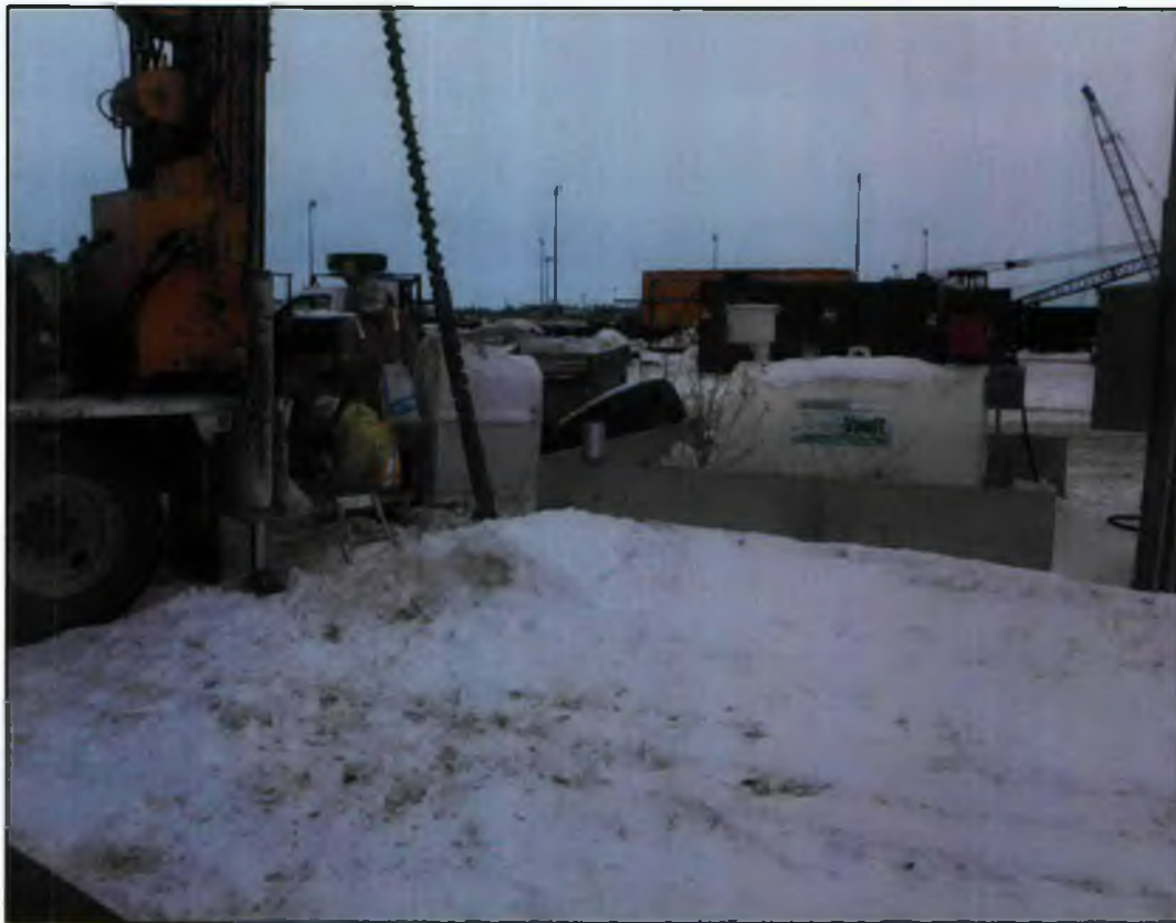
View looking north of the drill rig advancing BH04
