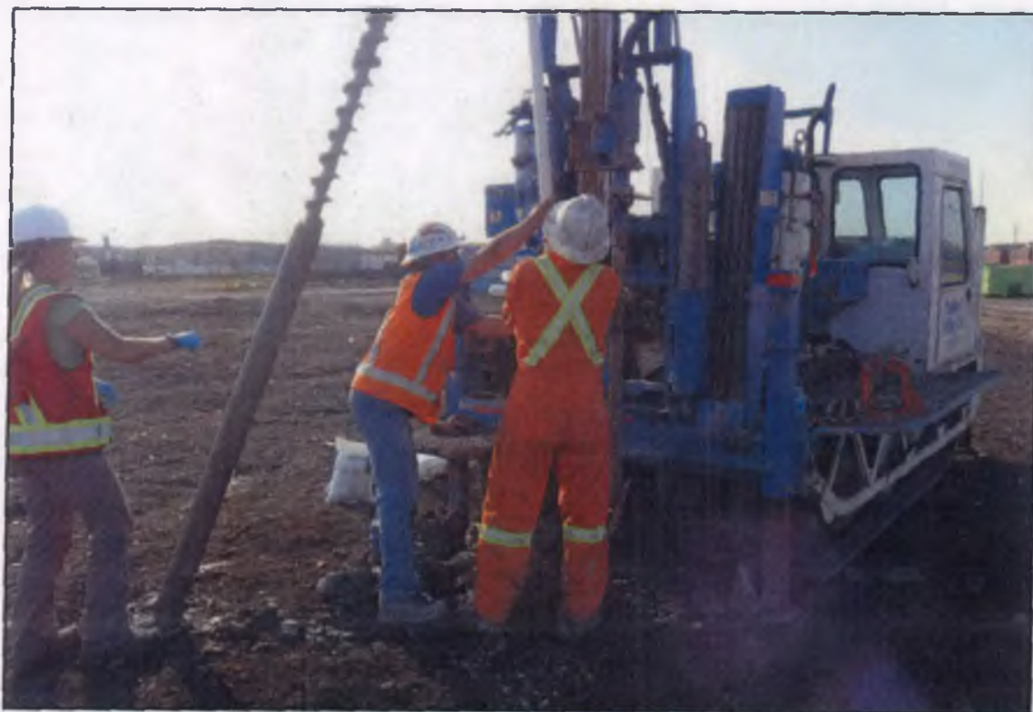
View of the installation of MW07 looking northeast.
