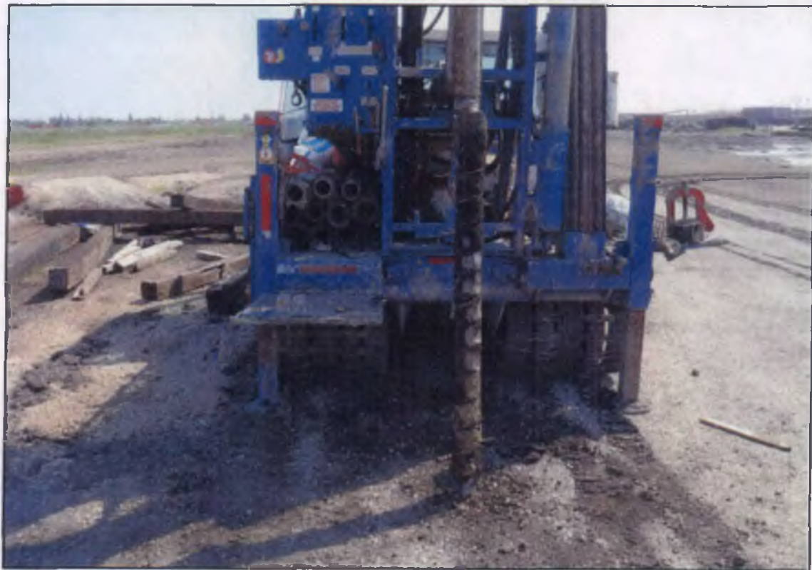
View of BH13 looking north.
