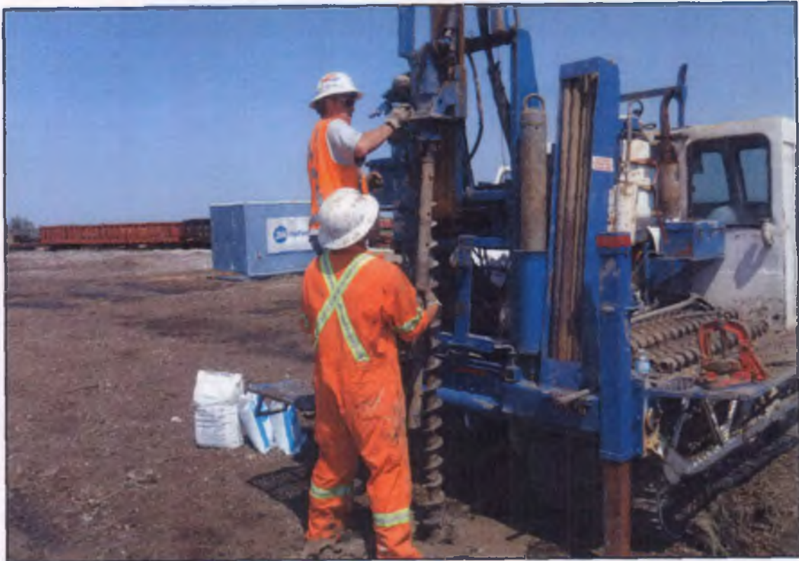
View of MW09 looking northwest.
