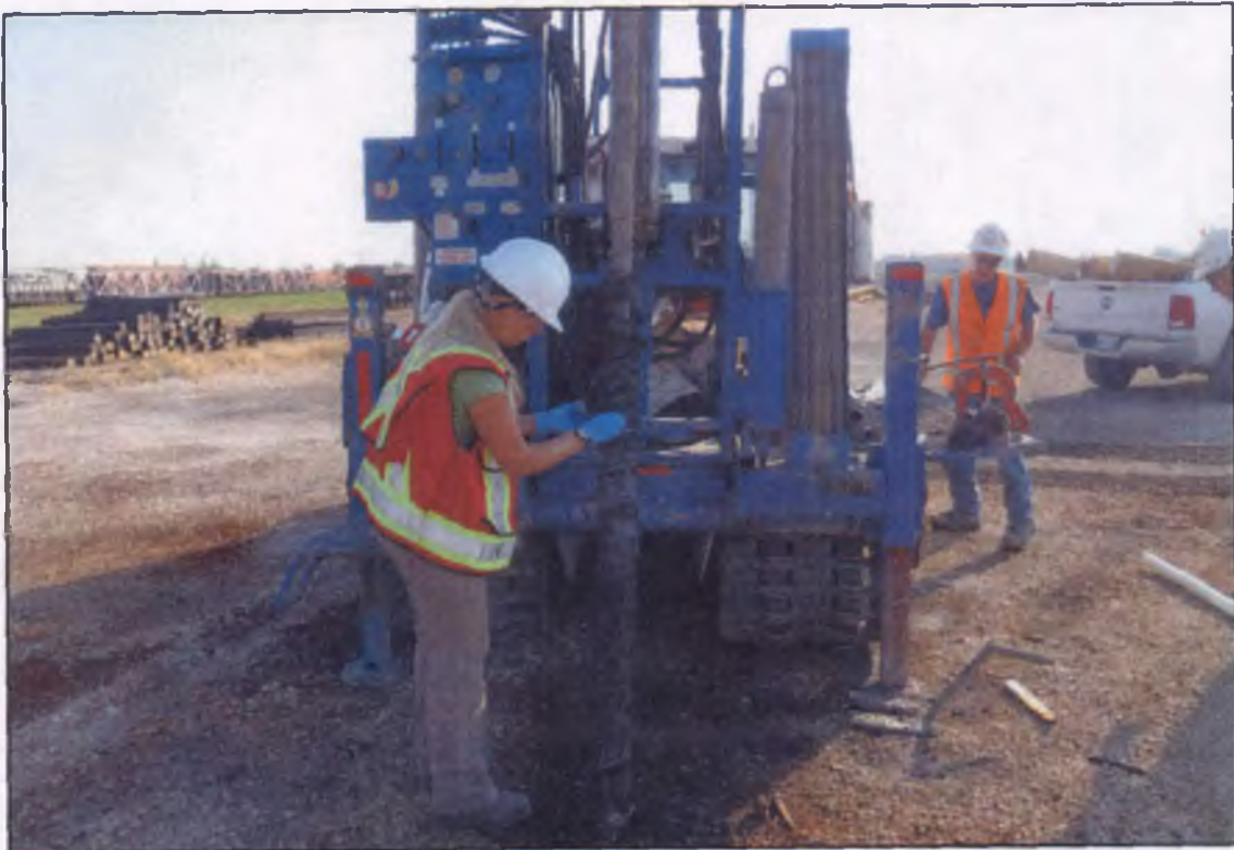
Sampling of MW01(MW10) looking northwest.
