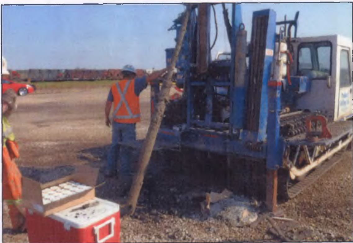
View of BH10 looking west.
