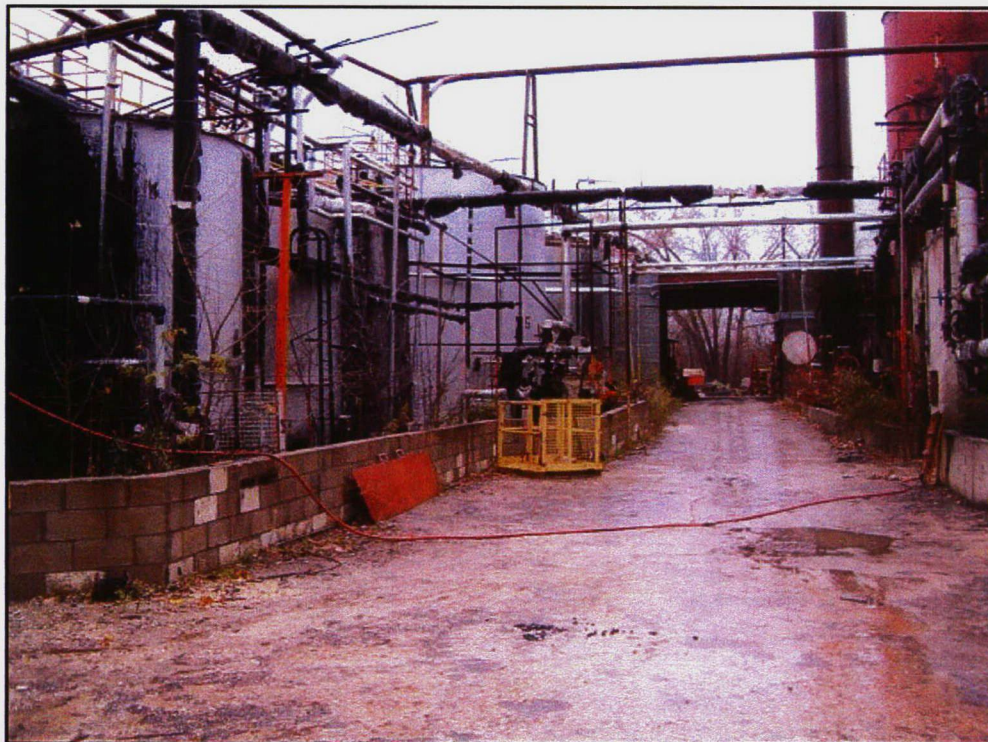
PHOTOGRAPH #44: View of asphalt tanks between Buildings J and E, facing south.
