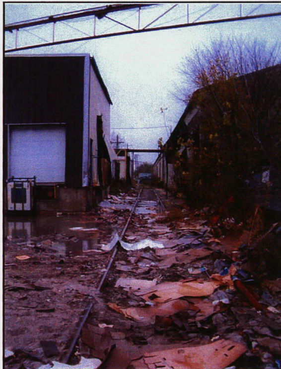
PHOTOGRAPH #25: View of a rail spur facing east.
