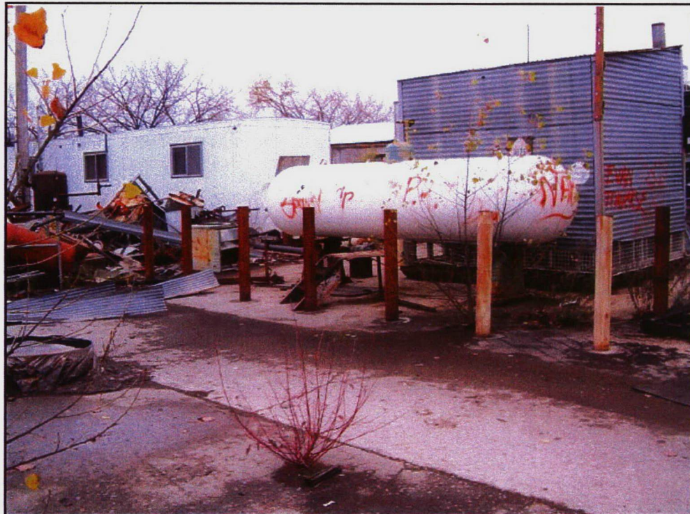
PHOTOGRAPH #46: View of a propane tank on the south side of Building J.
