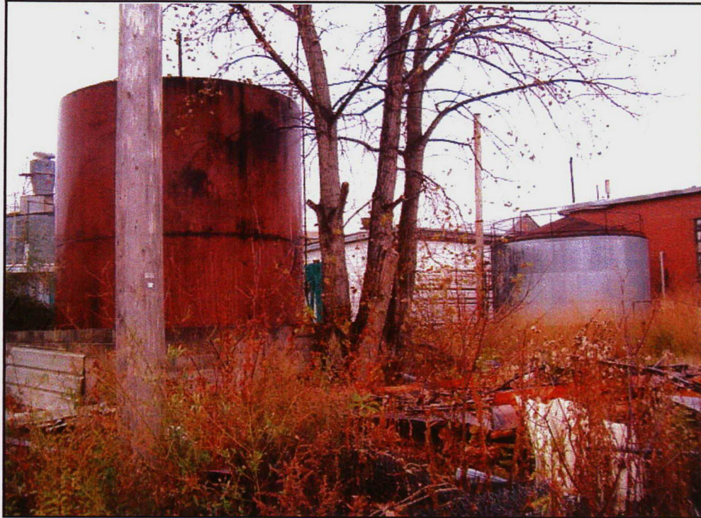
PHOTOGRAPH #45: View of a thermal oil tank on the left and an asphalt tank on the right.
