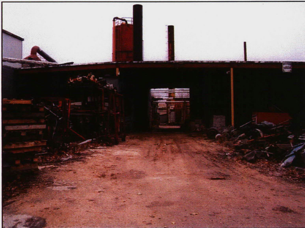
PHOTOGRAPH #12: View of causeway through Building H.
