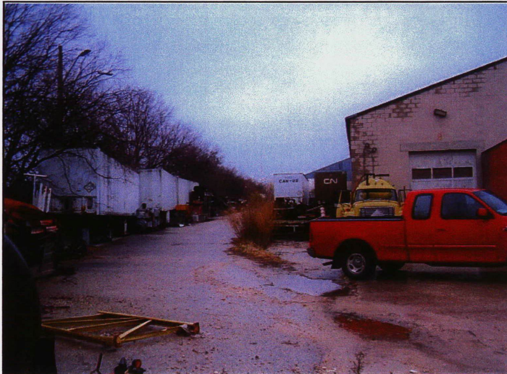
PHOTOGRAPH #27: View of metal storage along the north property line facing east.
