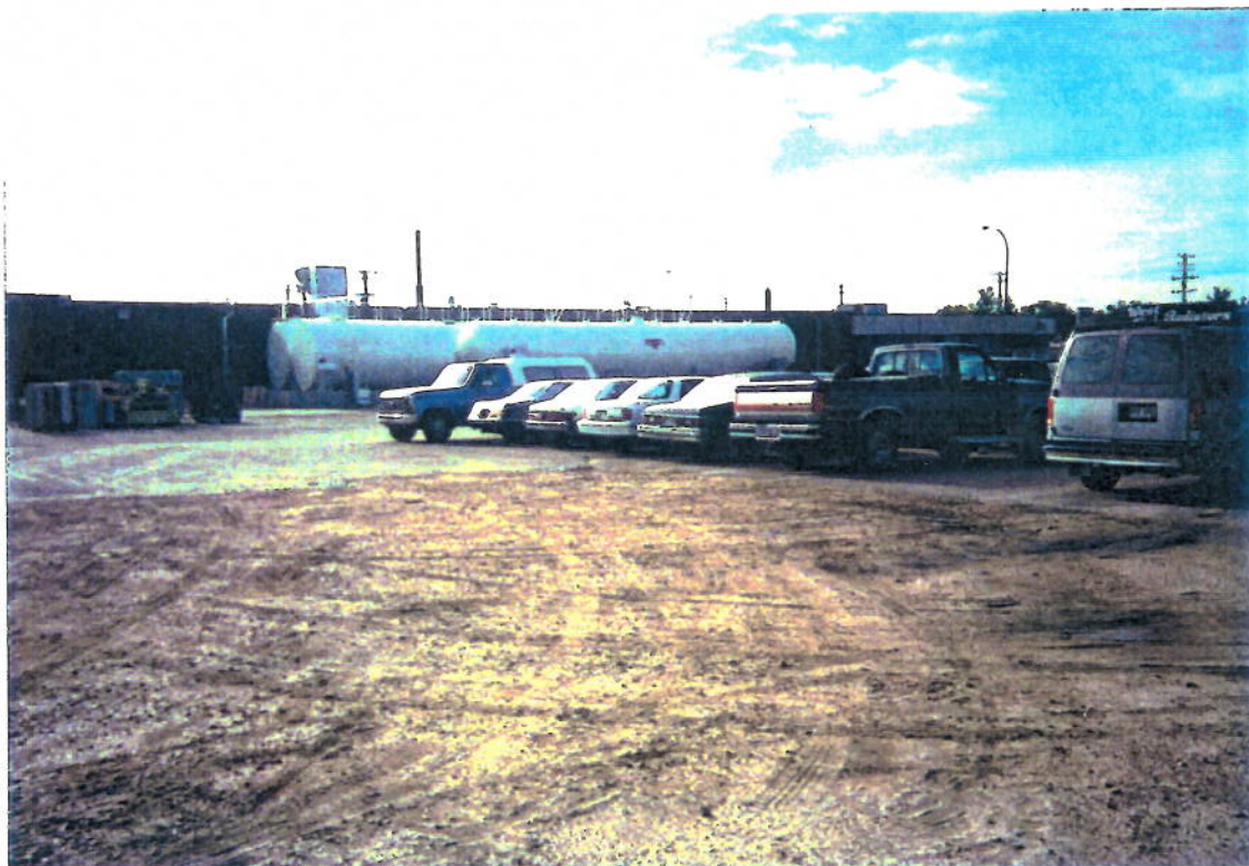
Photo 3 - View of tank compound and parking lot to the west of tank compound, looking southeast.
