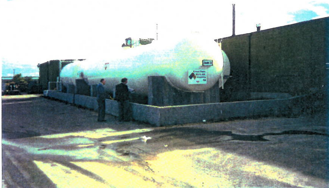
Photo 1 - View of tank compound looking northeast. MW-1 is located at south end of Tank 2. MW-4 is located at southeast corner of compound, at right of photograph.
