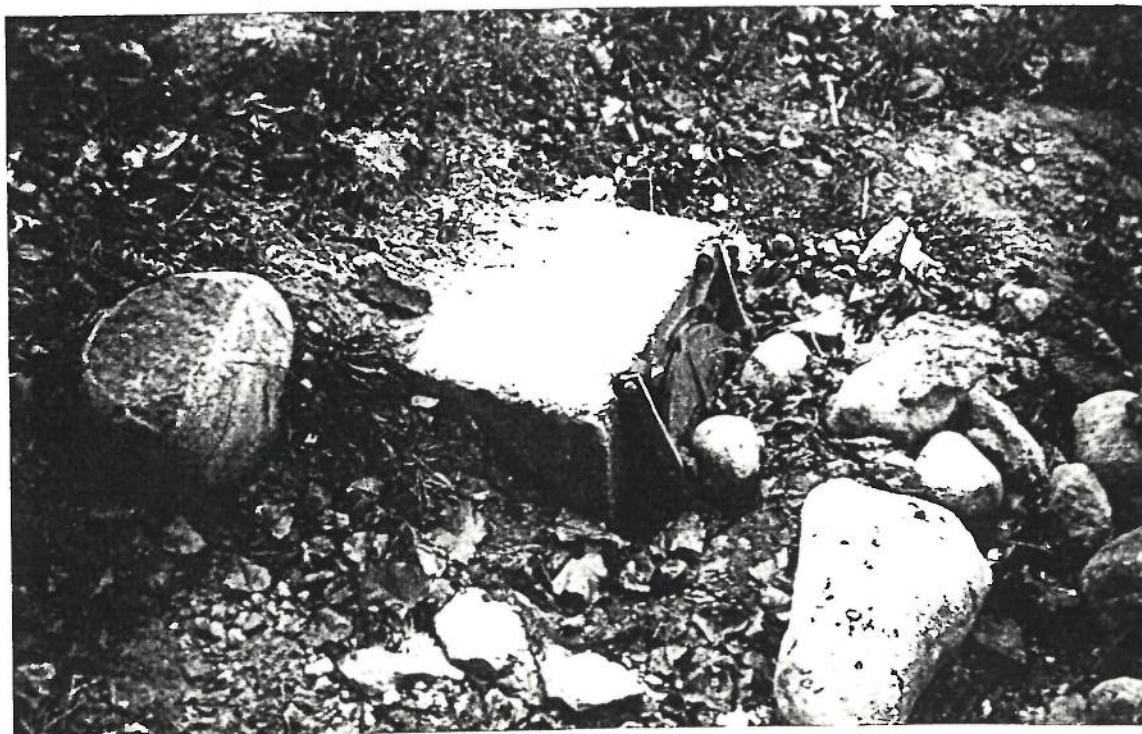
PHOTOGRAPH 2: Outfall from deck drains, west of the Disraeli Bridge abutment.
